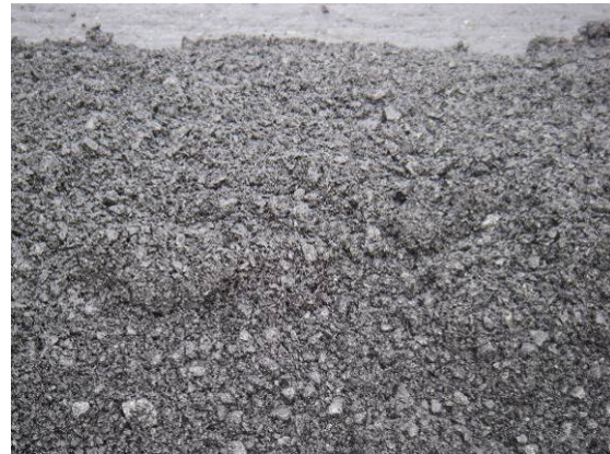
Figure 12. Clumps in windrow during placement of WMA on I-90.
