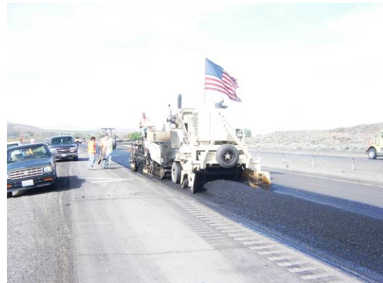
Figure 6. Windrow elevator picking up mix in windrow.
