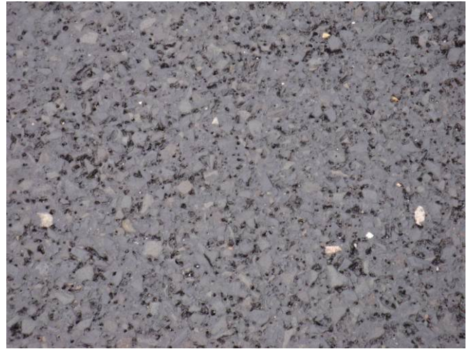
Figure 29. HMA section close-up. (Jan. 2011)
