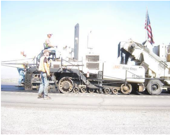
Figure 7. Windrow elevator delivering mix to machine.
