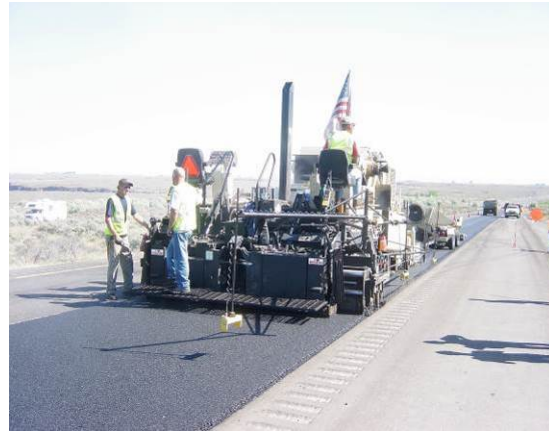
Figure 8. Paving machine spreading the mix.
