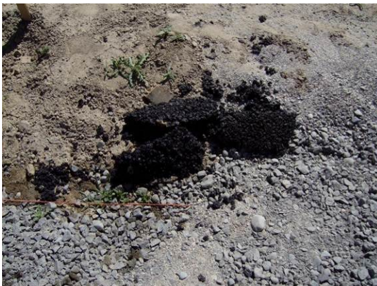
Figure 11. Clumps removed from WMA during test section near Quincy.
