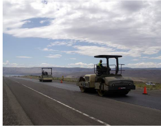
Figure 10. Breakdown and intermediate rollers.
