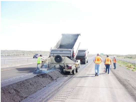
Figure 5. Truck dumping into the windrow device and forming windrow.
