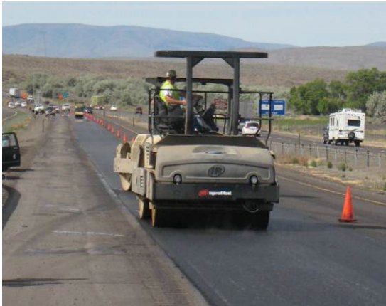
Figure 9. Breakdown roller.
