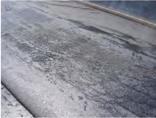
Figure 16. Mix pickup area immediately after rolling.
