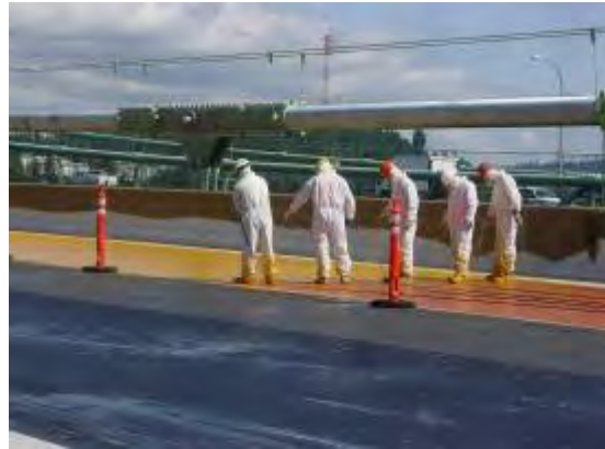
Figure 8. Applying methyl methacrylate isolation layer.
