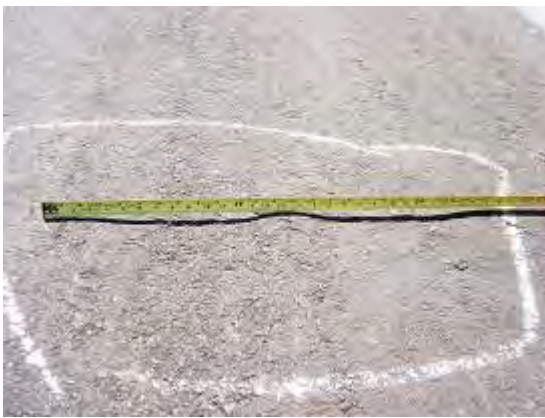
Figure 39. Tire indentation near west end.
