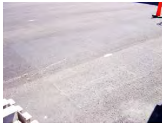
Figure 40. Indentation left by Demag crane pad.
