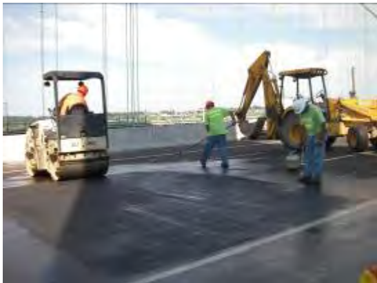
Figure 48. Finished conventional HMA patch.
