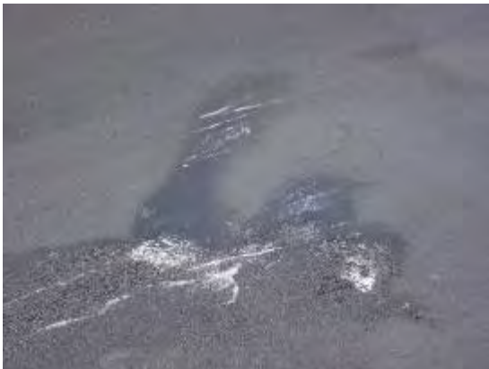
Figure 18. Area of mix pickup after completion of rolling.
