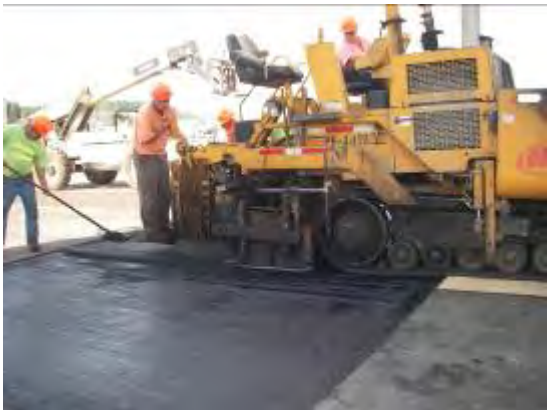
Figure 47. Replacing top course with conventional HMA.
