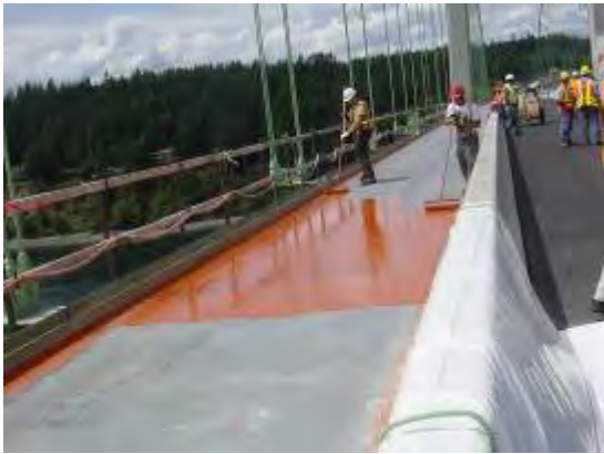
Figure 7. Applying acrylic based prime coat bonding layer.
