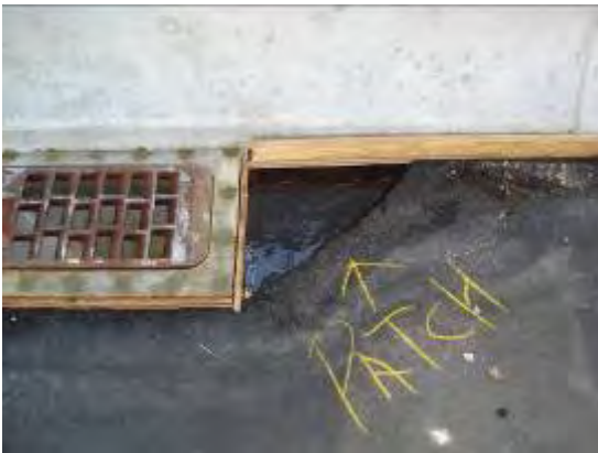
Figure 24. Adhesion layer repaired.
