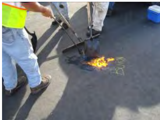
Figure 38. Repairing indentation.
