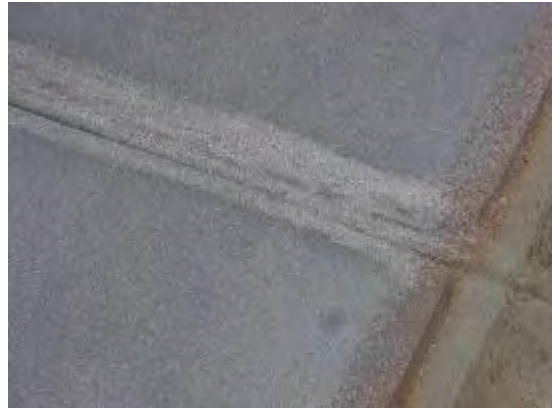
Figure 6. Steel deck after shotblasting.
