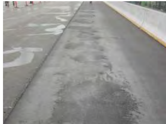
Figure 19. Area of mix pickup prior to the next day's paving.
