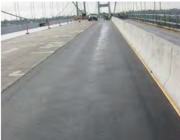
Figure 31. Steaks in base course on Lane 1.
