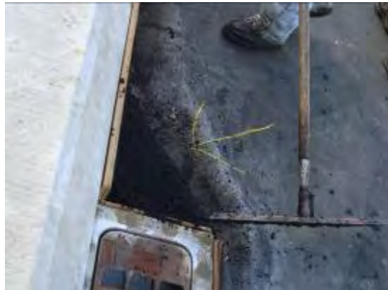
Figure 25. Repaired adhesion layer.
