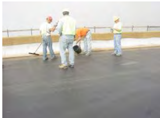
Figure 10. Repairing adhesion layer.
