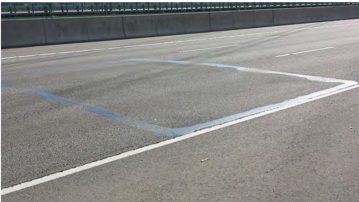
Figure 61. Patch Lane 1 and 2. Patch was done in July 2007 to repair problems caused by a solvent spill on the original overlay. Patch material was conventional HMA. (Photos from 5/1/14)
