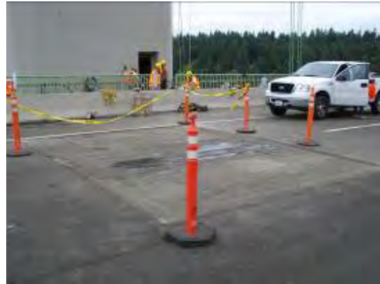
Figure 44. Damaged pavement removed from Lane 2 and 3.
