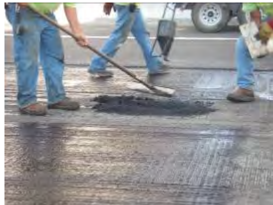
Figure 46. Repairing base course with conventional HMA.
