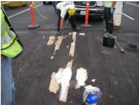
Figure 45. Repairing isolation layer.
