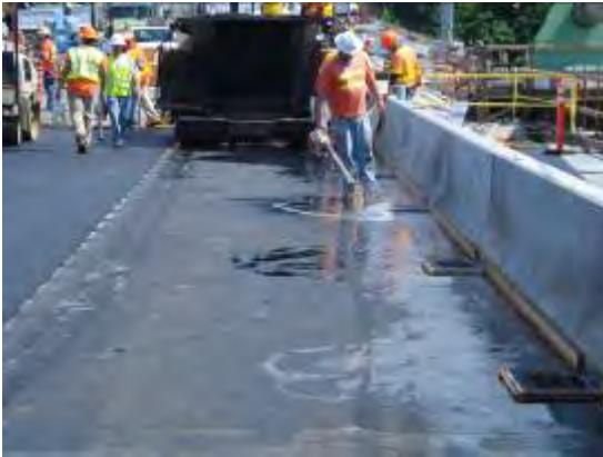
Figure 22. Water being removed prior to paving.
