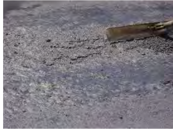
Figure 17. Raking in mix to repair pickup area.
