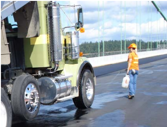
Figure 20. Applying water to prevent damage to adhesion layer.
