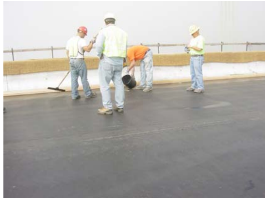
Figure 8. Repairing adhesion layer.
