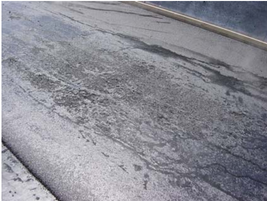
Figure 16. Mix pickup area immediately after rolling.
