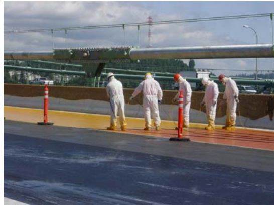
Figure 6. Applying methyl methacrylate isolation layer.
