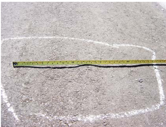
Figure 39. Tire indentation near west end.
