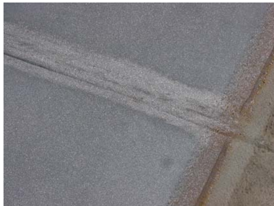
Figure 4. Steel deck after shotblasting.
