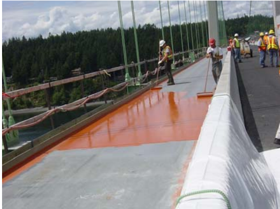
Figure 5. Applying acrylic based prime coat bonding layer.
