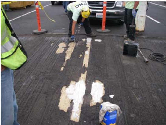
Figure 45. Repairing isolation layer.
