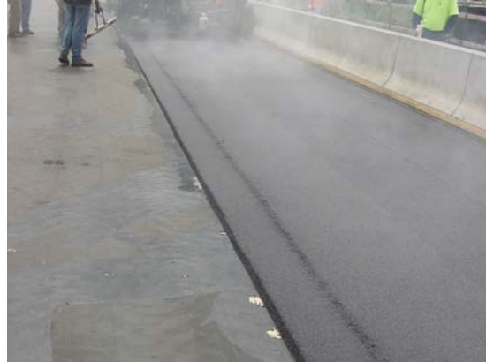
Figure 34. Streak left by screed extension.
