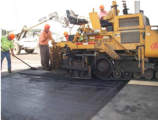
Figure 47. Replacing top course.
