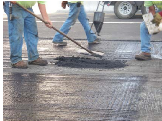
Figure 46. Repairing base course.
