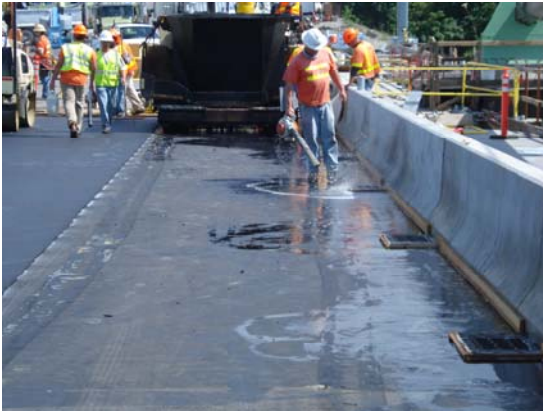
Figure 22. Water being removed prior to paving.
