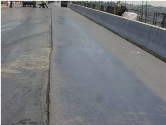
Figure 35. Flushing in lane one immediately after paving.
