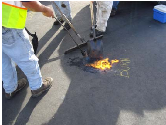
Figure 38. Repairing indentation.
