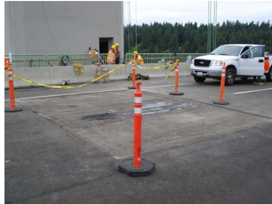
Figure 44. Damaged pavement removed from lane 2 and 3.
