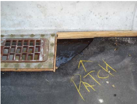
Figure 24. Adhesion layer repaired.
