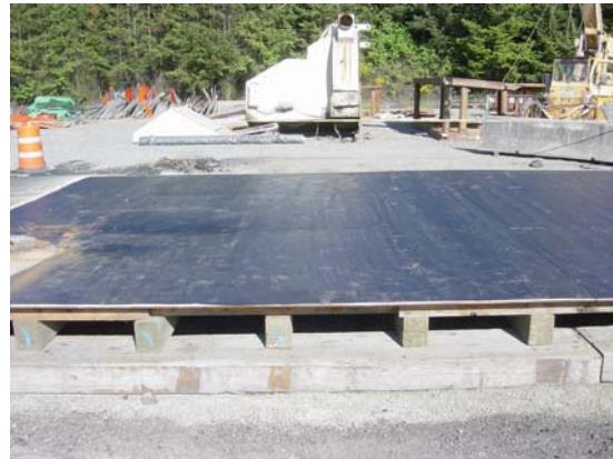
Figure 14. Simulated orthotropic bridge deck.
