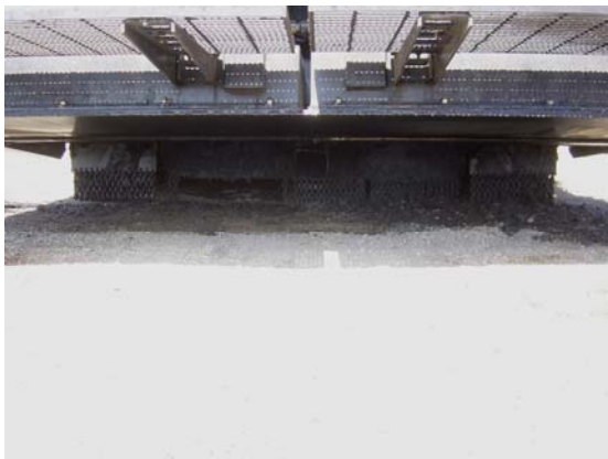
Figure 11. Missing chains on MMK retrofit on Ingersoll-Rand Blaw-Knox PF-4410 paver.
