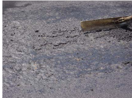
Figure 17. Raking in mix to repair pickup area.
