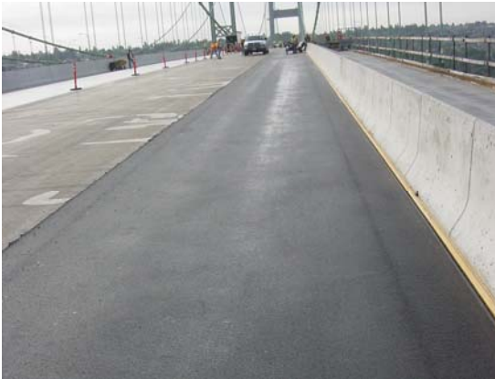
Figure 31. Steaks in base course on lane one.
