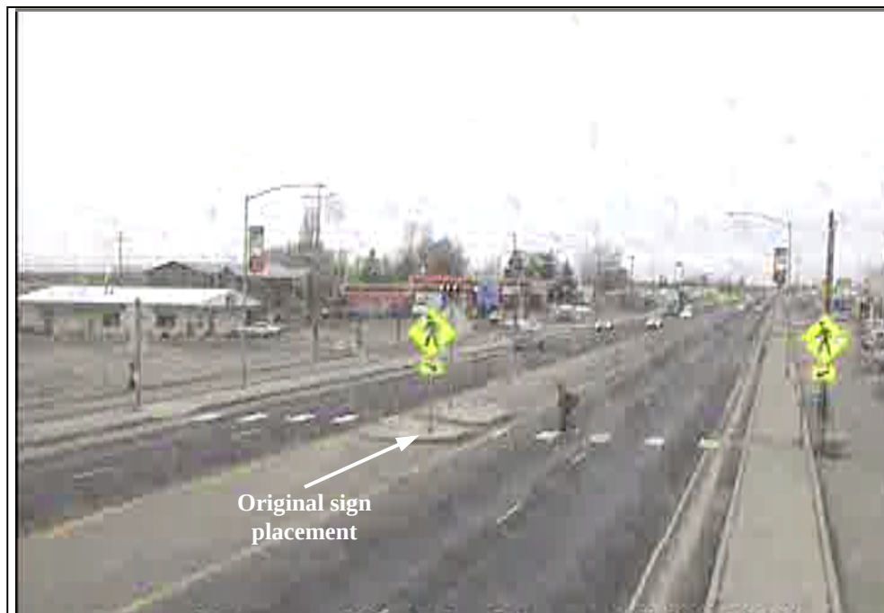
Figure 3.9. Median sign placement— before condition—Airway Heights
