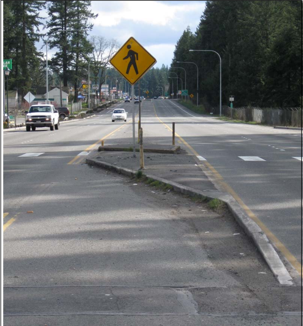
Figure 3.3. Front view of median with crosswalk markings—Spanaway
