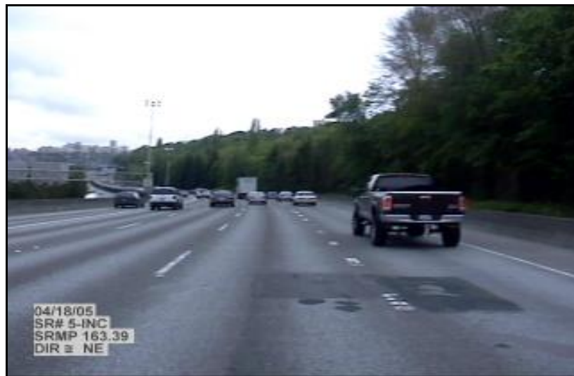
Figure 3. Photo Log from WSDOT of Pavement Around Spokane St.
