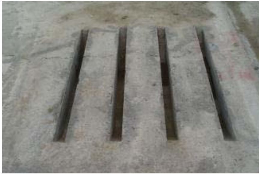
Figure 4.1. Dowel Bar Slots (Image Courtesy Pavement Interactive)
