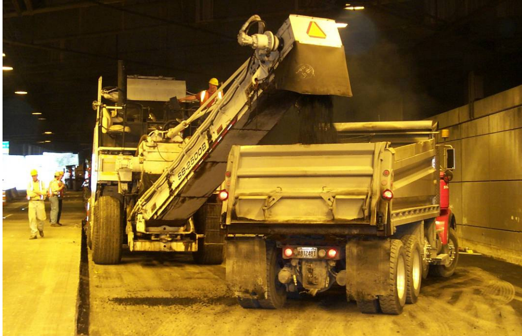
Figure 19 - HMA material transfer vehicle loading HMA truck in the construction pit (Photo courtesy of WSDOT).
