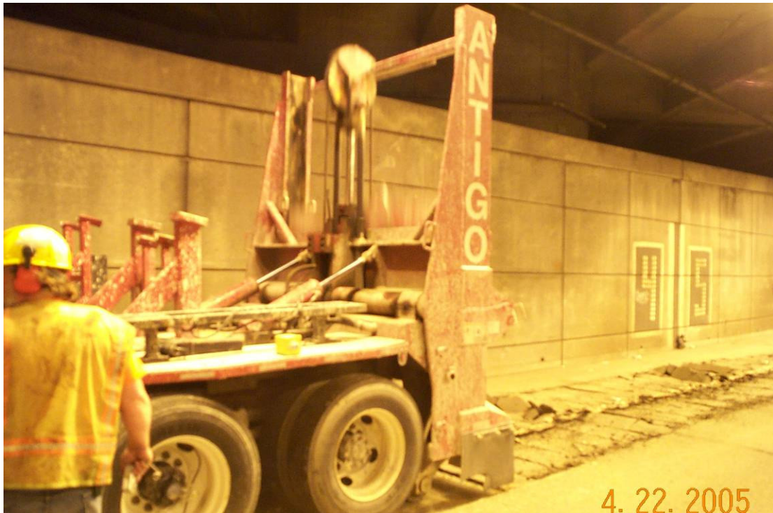
Figure 9 - Truck mounted drop hammer breaking PCC pavement under the Washington State trade and Convention Center (Photo courtesy of WSDOT).
