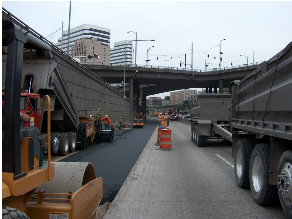
Figure 12 - Delivery, placement and compaction of HMA pavement with one access lane (Photo courtesy of WSDOT).
