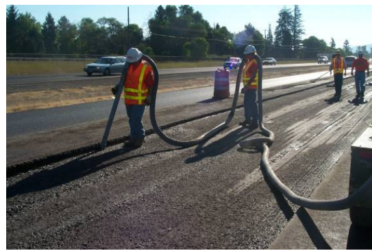
Image B. Cleaning of the existing pavement surface. Note remnants of the Superpave overlay in the wheelpaths.
