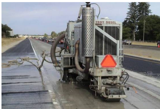
Image E. Diamond grinding to remove the ruts from the vehicle that entered the construction zone.
