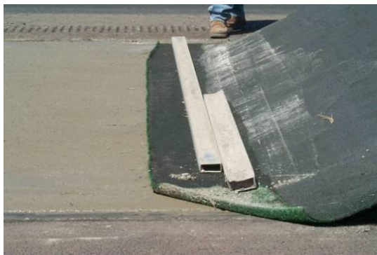
Image E. Close-up of weights use to keep the carpet in contact with the wet concrete.
