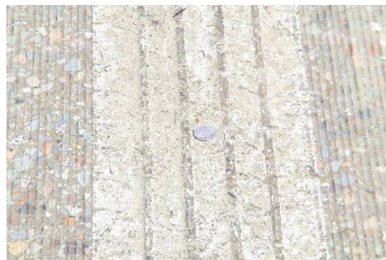
Image F. Ruts caused by vehicle that entered the construction zone during paving.
