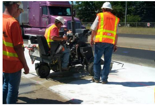
Image B. Joint sawing operation.
