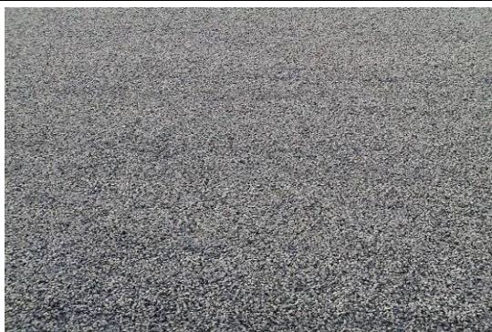
Image E. Completed macro-surfacing overlay.
