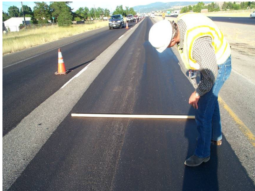
Figure 8. Micro-surfacing placed as a rut fill prior to macro-surfacing within the two westbound lanes of I-90 (MP 293.15 to MP 293.55).
