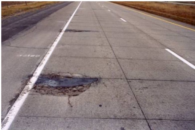
Figure 22. Cracking in MnROAD Test Cell 95, 3 inch whitetopping with a 5 ft by 6 ft joint spacing. Photo courtesy of Mn/DOT.
