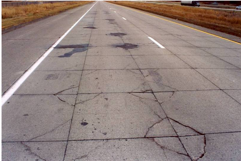
Figure 21. Corner cracking in MnROAD Test Cell 94, 3 inch whitetopping with a 4 ft by 4 ft joint spacing. Photo courtesy of Mn/DOT.
