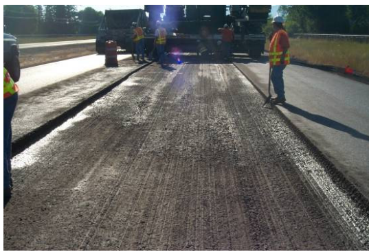
Image A. Existing pavement after grinding operation. Note remnants of the Superpave overlay in the wheelpaths.
