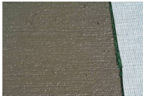
Image F. The finished texture after the carpet drag.
