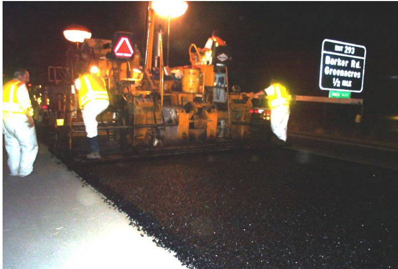
Figure 5. Paving of Modified Class D mix.
