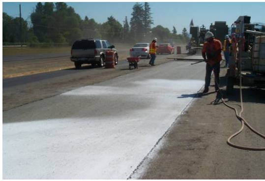
Image A. Hand application of curing compound.
