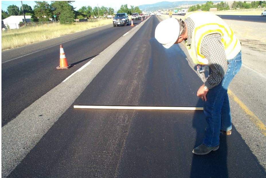
Image 3. Micro Surfacing placed as a rut fill prior to Macro-Surfacing within the two westbound lanes of I-90 (MP 293.15 to MP 293.55).
