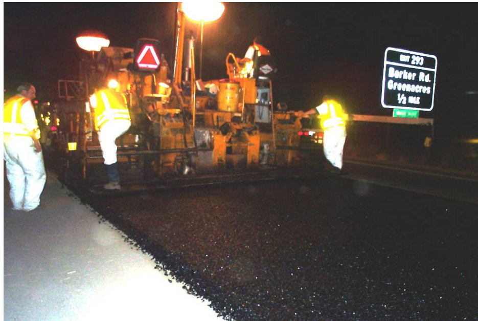
Image 2. Placement of Modified D asphalt in the inside eastbound lane of I-90 (MP 293.15 to MP 293.55).
