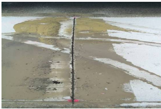
Image C. Spalling of joints due to tender mix or fibers or a combination of both.
