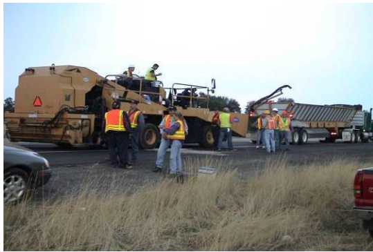
Image A. Paving train for macro-surfacing.
