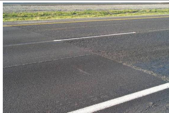
Image F. Macro-surfacing overlay on the right and existing pavement on the left.
