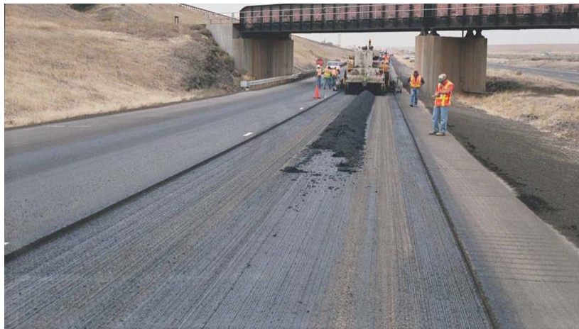
Figure 2.1: Tracking due to the presence of debris.
