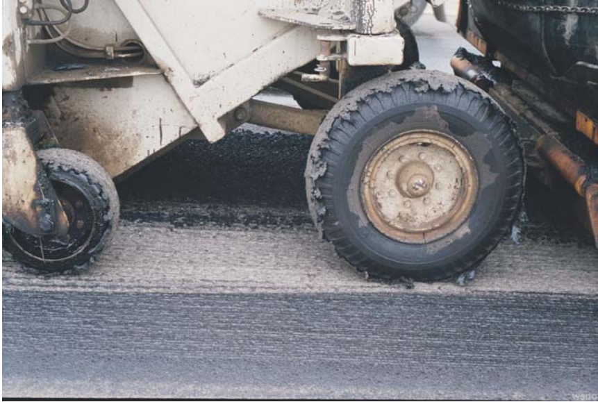
Figure 10: Tracking as seen on separate WSDOT HMA paving projects.
