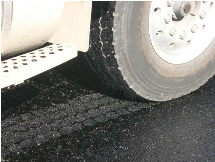
Figure 3.11: Equipment tracking during this experiment.
