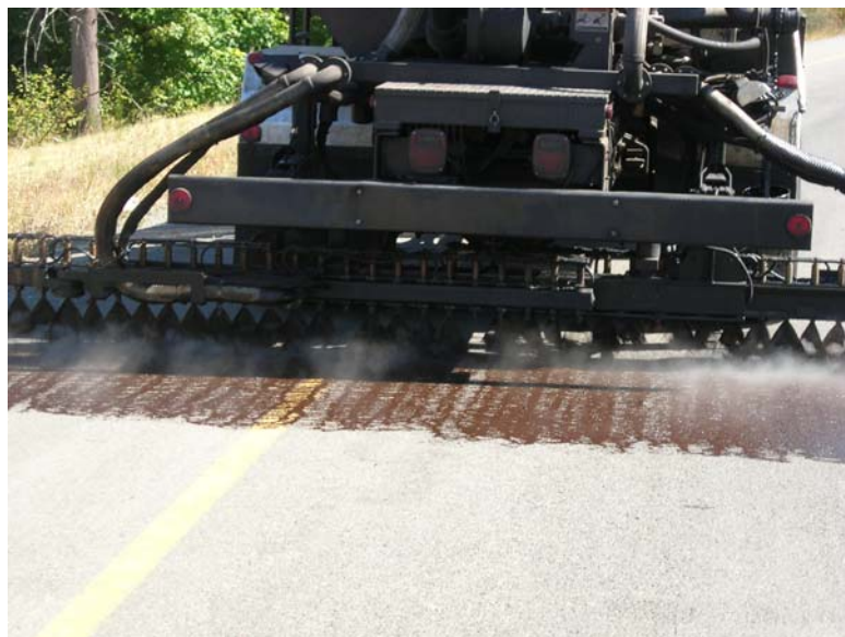
Figure 1.1: A truck spraying tack coat on an HMA surface.
