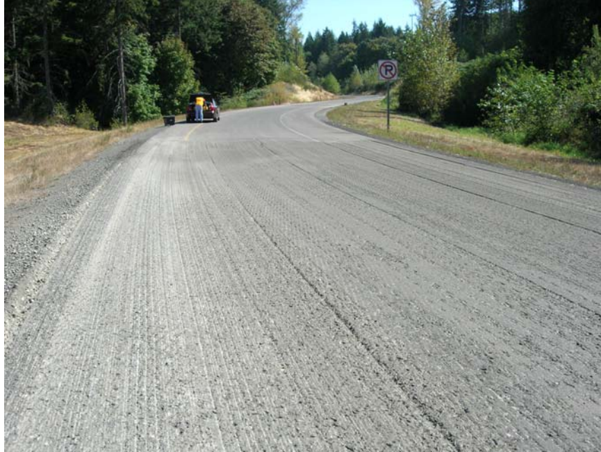
Figure 3.2: Milled and non-milled sections after cleaning.
