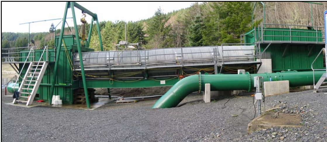
Figure 40. Culvert at 4.3% Slope
