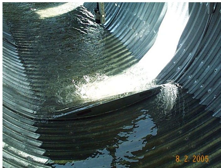
Figure 2. Washington Department of Fish and Wildlife Culvert-Retrofit Baffle Installation
