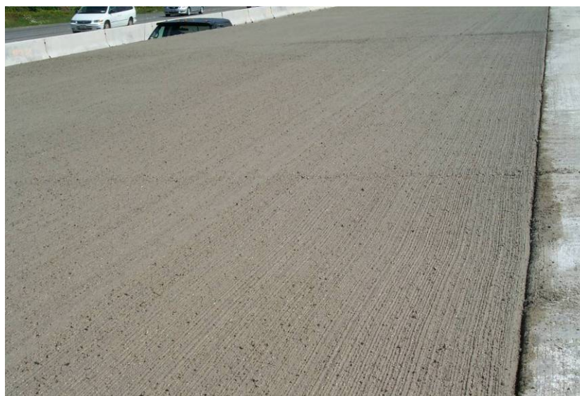
Figure 18. Carpet drag texture on the I-5 Pierce Co. Line Project.
