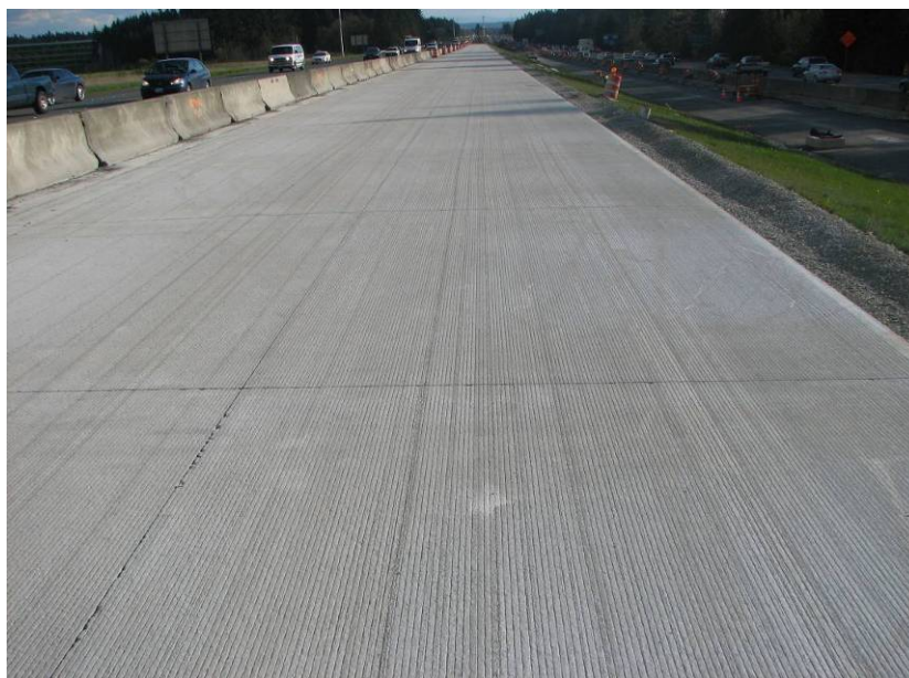
Figure 19. Longitudinal tining on the I-5 Pierce Co. Line Project.
