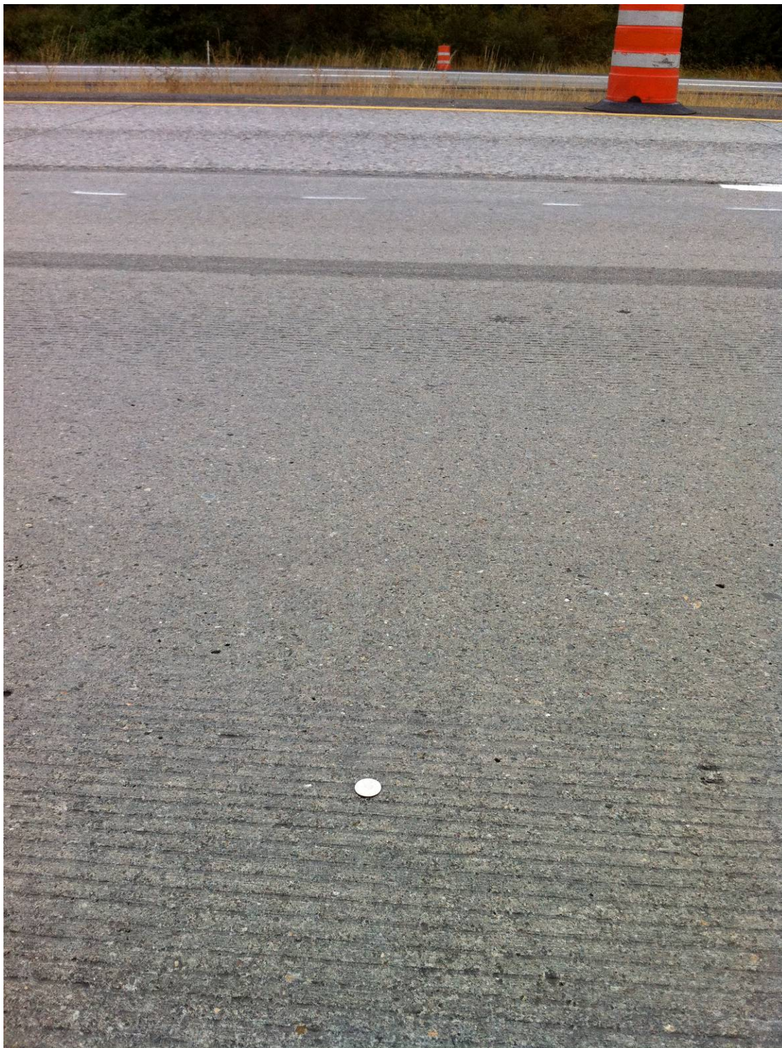
Figure 14. Example of rapid wear from studded tires on a longitudinal tined pavement on I-90 near Cle Elum. Photo taken after one winter of wear.
