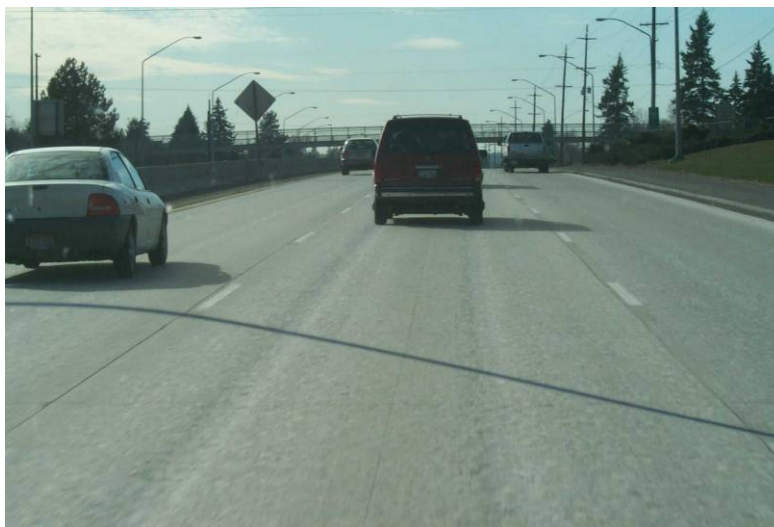
Figure 3. Studded tire wear on a concrete pavement (I-90 Spokane).
