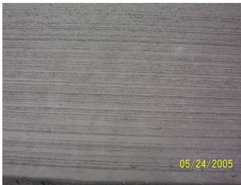
Figure 16. Carpet drag texture on the I-5 Federal Way Project immediately after construction.
