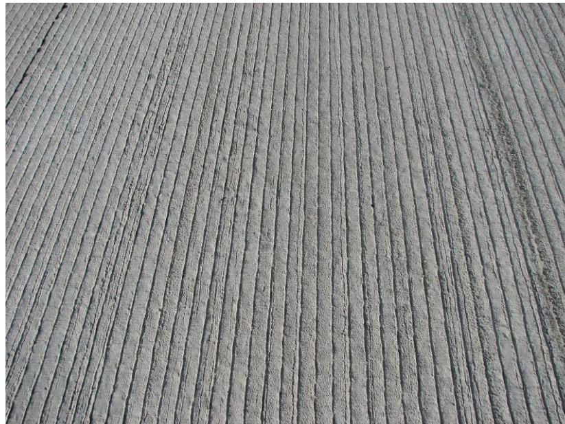
Figure 20. Close-up of the longitudinal tining on the I-5 Pierce Co. Line Project.
