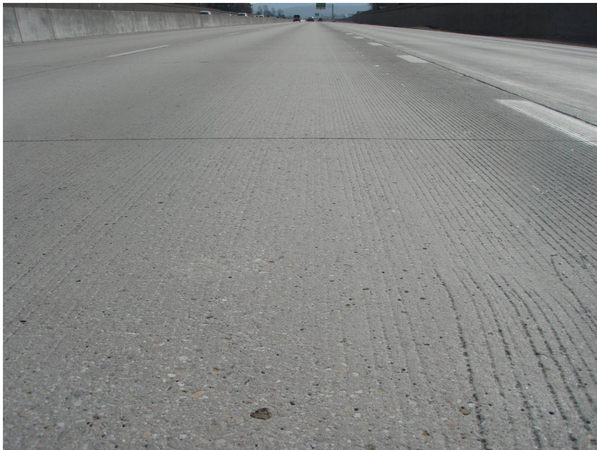
Figure 13. Example of rapid wear from studded tires on a longitudinal tined pavement on I-90, Sullivan to Barker, paved in 2011. Photo taken on 4/11/2012 after one winter of traffic.
