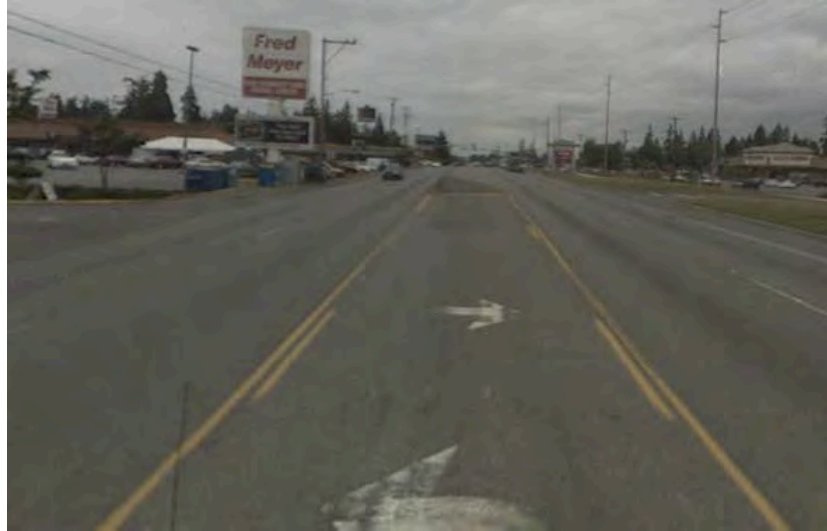
Figure 1: Example of a Two-Way Left Turn Lane (TWLTL) with Limited Access Control 1
