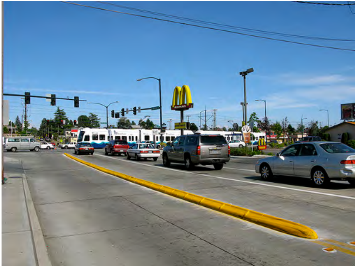
Figure 2: Example of a C-Curb 2 Separating Directions of Traffic
