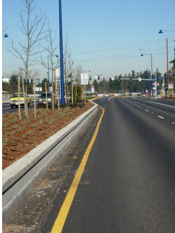
Figure 5: Des Moines Median Treatment: Trees Behind a Low Profile Barrier 23
