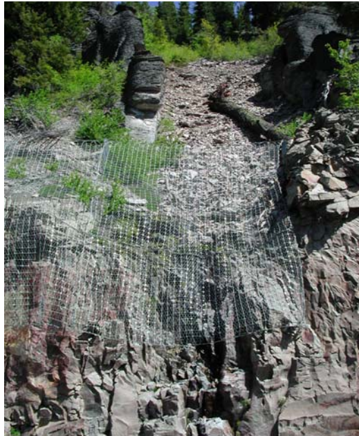
Figure 5-8. Modified cable net installation, upslope source of rockfall, and typical range of block sizes that impact the installation in a sub-perpendicular orientation.
