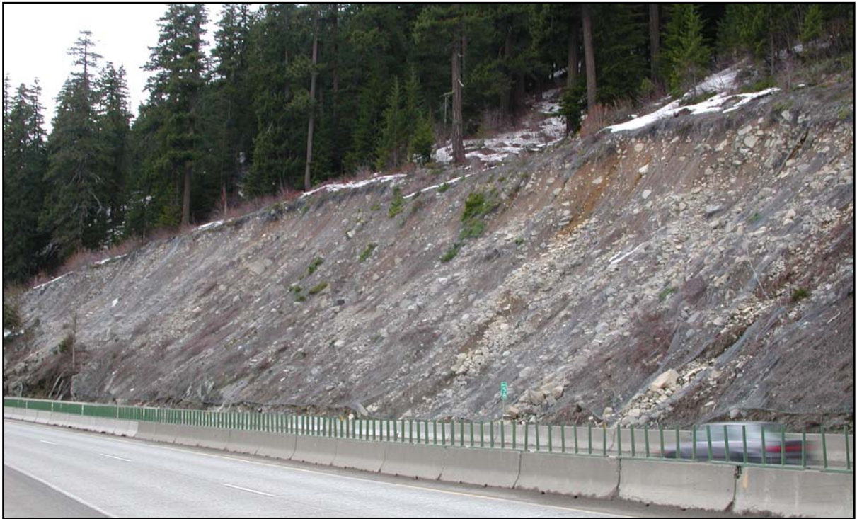
Figure 2-8. Looking west of the West Snowshed slope, active raveling near the crest of the cut slope and a large percentage of boulders within the debris.
