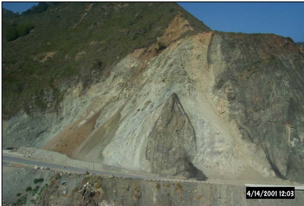
Figure 2-4. Slope condition after slope instabilities destroyed the hexagonal wire mesh installation at Pitkins Curve adjacent to Rain Rocks chute.
