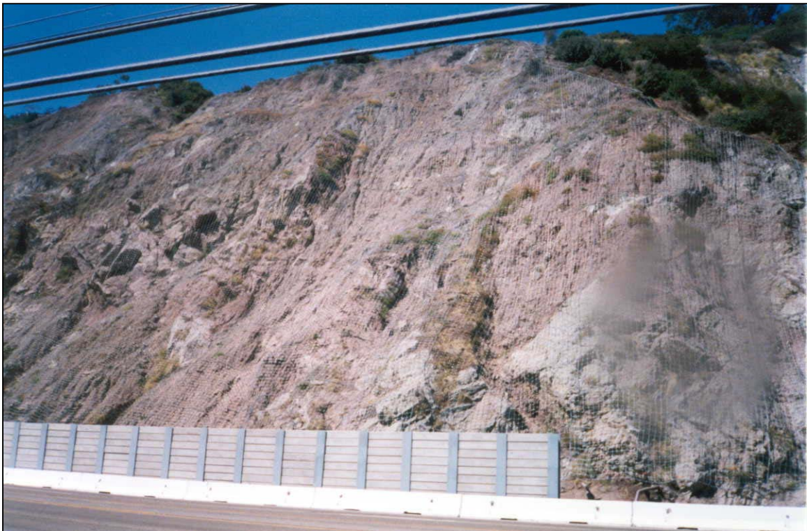
Figure 2-2. Slope condition after the slope was covered with a cable net.
