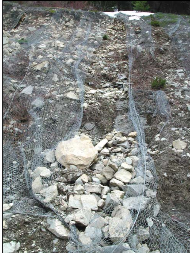
Figure 2-10. Rupture of the vertical seam and fabric; the midslope horizontal support cable was also damaged. The volume of debris associated with mesh failure is estimated to be 10 cubic yards, with block sizes of up to 3.5 feet in dimension.
