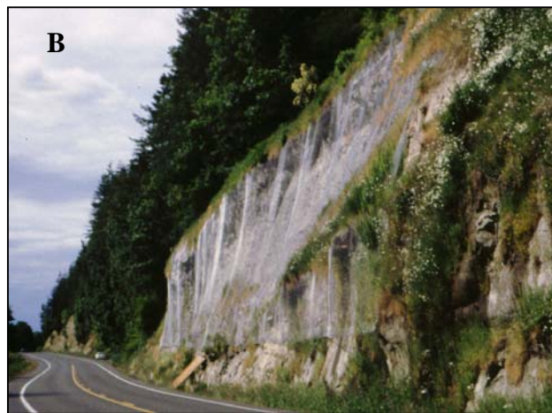
Figure 7-9. (A) The mesh was carefully installed to closely conform to this moderately inclined slope. (B) On a steep to overhanging slope where mesh conformance is generally more difficult to achieve, the mesh can become more visually apparent.
