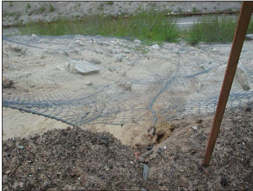
Figure 4-15. View looking downslope; note numerous boulders protruding into the mesh. With the exception of the top, where erosion has partially undermined the installation, the mesh is largely in contact with the slope.
