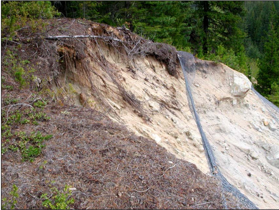
Figure 7-3. Ongoing erosion threatens a wire mesh system installed in the late 1980s in the North Cascades of Washington.
