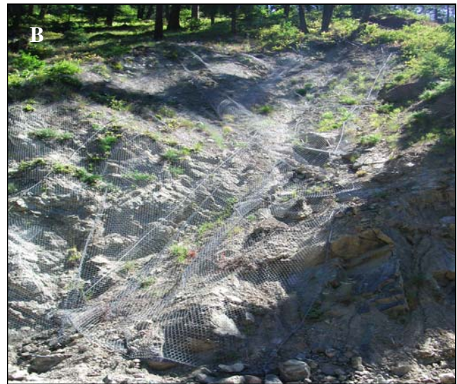
Figure 4-9. Slope area in (A) 1997 before and (B) 2002 five years after mesh installation and just after repair of the system.
