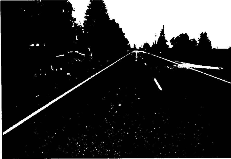
Figure 4.43 - Location of test pit and condition of roadway, Rocky Butte to Bridgeport Bar.
