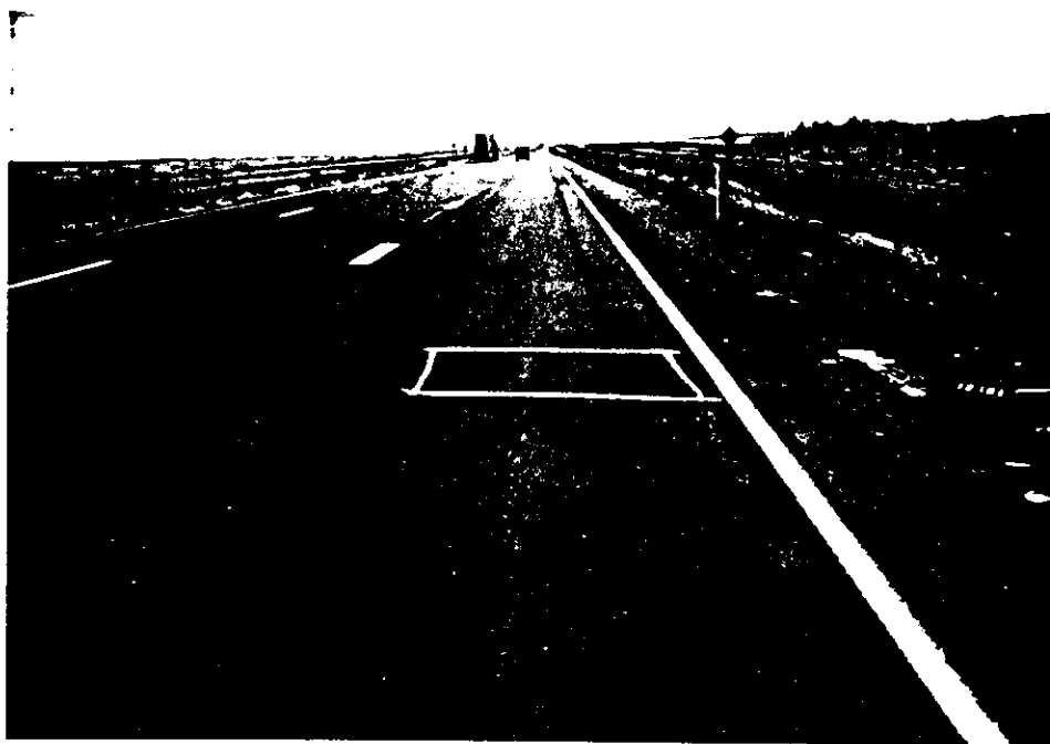
Figure 4.27 - Test pit location and condition of roadway, Ritzville to Tokio.
