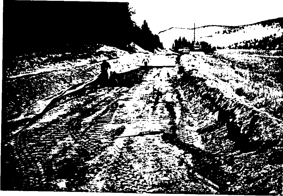
Figure 4.33 - Placing geotextile at Station 1131 to 1133 during construction, 6/15/89, Aeneas Valley Road to Wauconda Summit (courtesy S. Moore, WSDOT)
