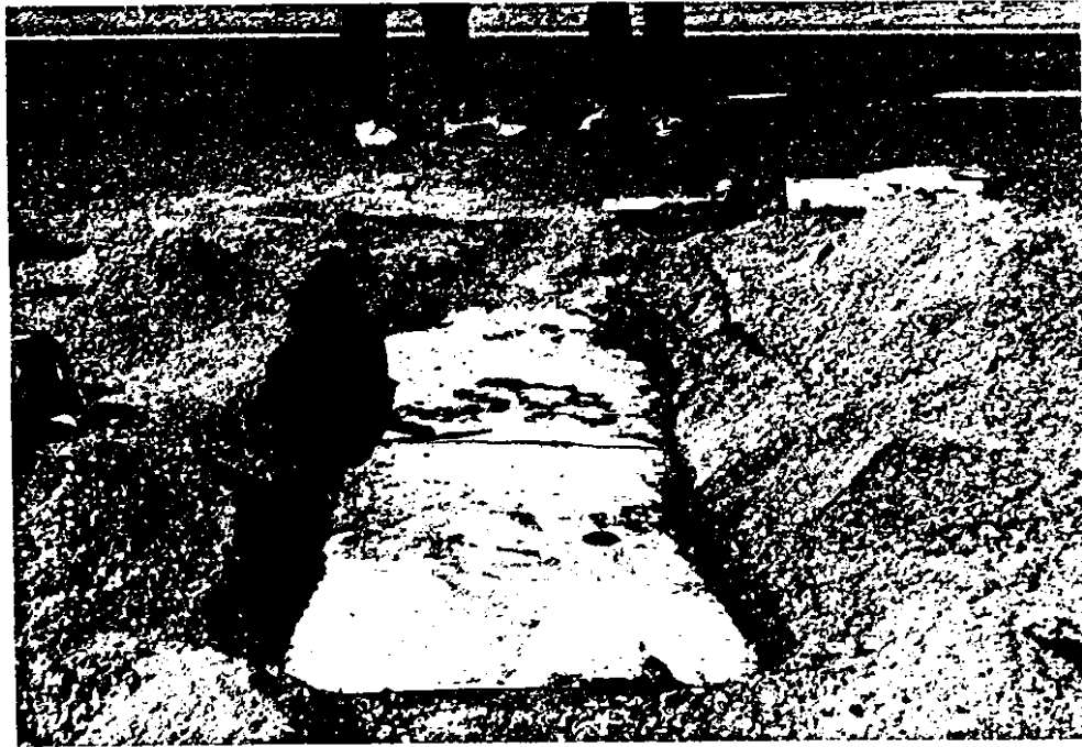
Figure 4.50 - Test pit showing shallow depth to geotextile, SR2/Farmer to 5NW Road.
