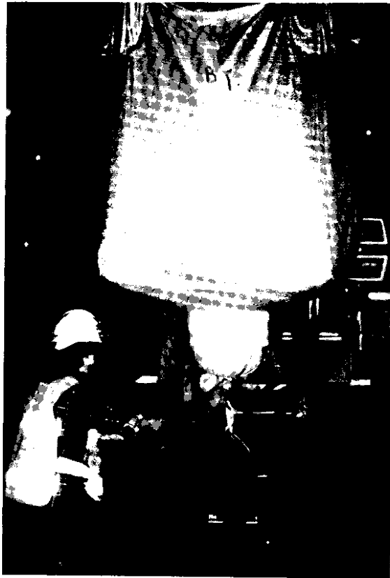
Dispensing aggregate to wheelbarrow.
