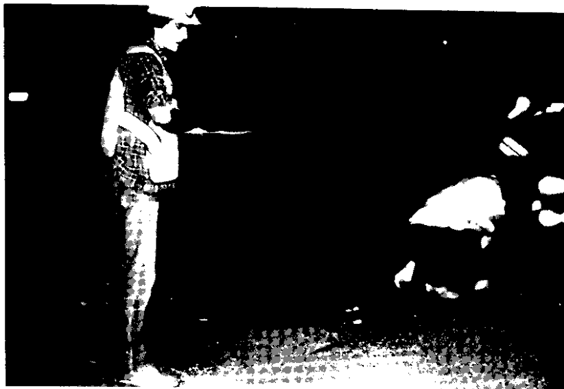
Spreading aggregate by hand from a hand shovel.
