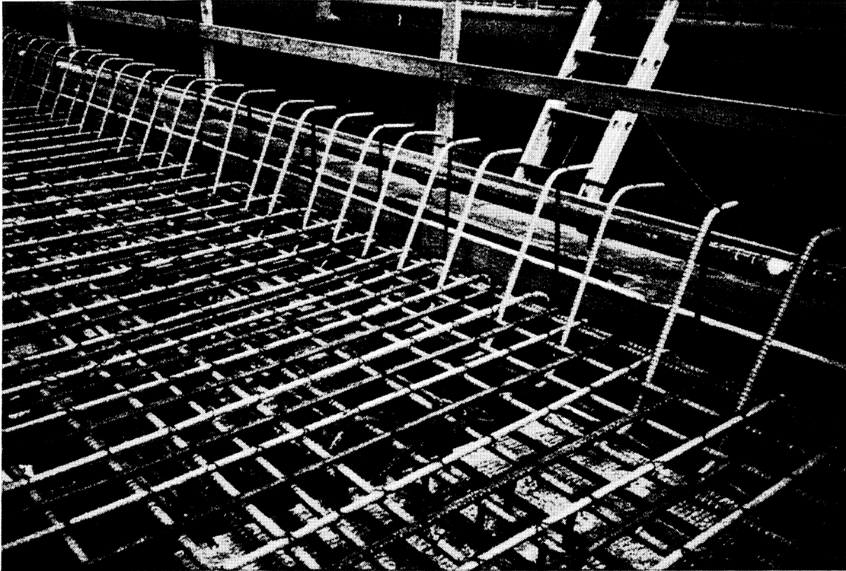
Figure 4.18 Field Test - Reinforcement in the Roadway Slab (portion of it can be seen)
