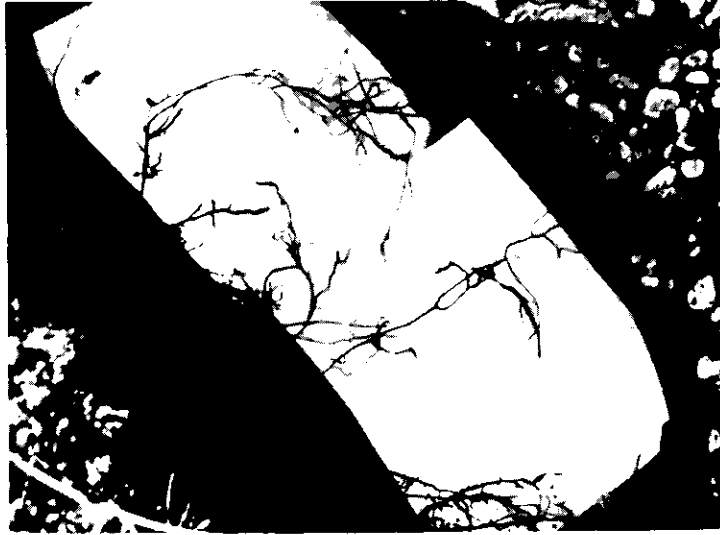
Figure 5 ROOTS FOUND IN GRAVEL BLANKET
