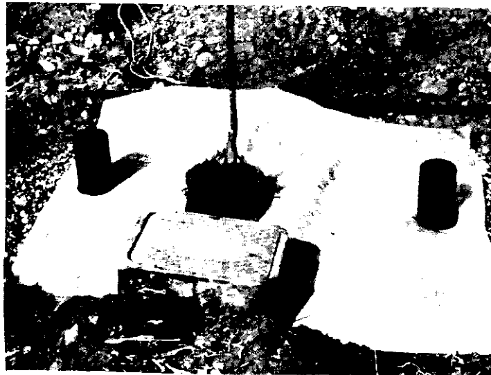
Figure 15 PLASTIC SLEEVES PLACED OVER RISERS
