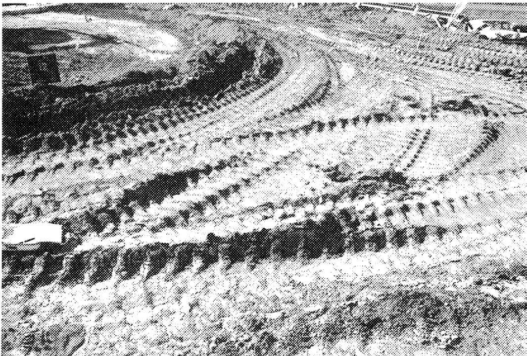
FIGURE 10. THIS SHOWS THE APPEARANCE OF THE SUBGRADE AFTER RING #2 PAVEMENT WAS REMOVED. NOTE THE TIRE TRACKS INDICATING THE SATURATED CONDITION OF THE PALOUSE SILT.
