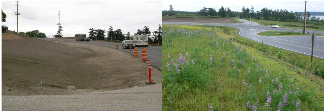
A before and after view of a meandering bioswale graded to blend into its surroundings.
