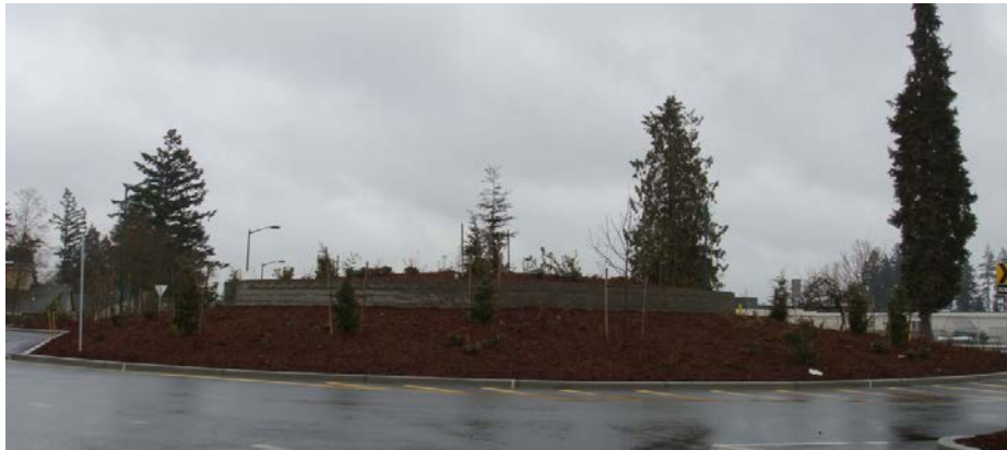
Mounding within the center of a low speed roundabout.
