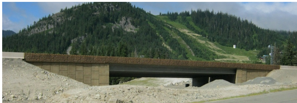
Continuity is enhanced by maintaining a single architectural theme throughout the corridor.
