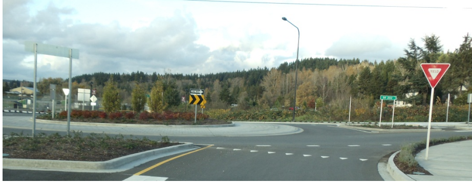
Low-growing groundcovers outside the roundabout, with trees and low shrubs within the roundabout.
