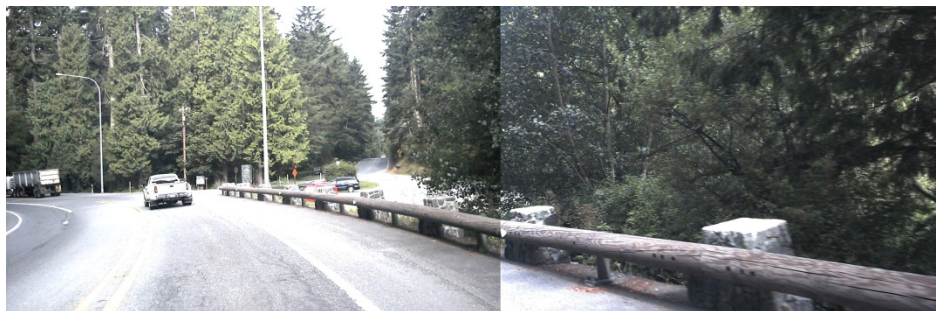
New guardrail is designed to blend with existing guardrail.
