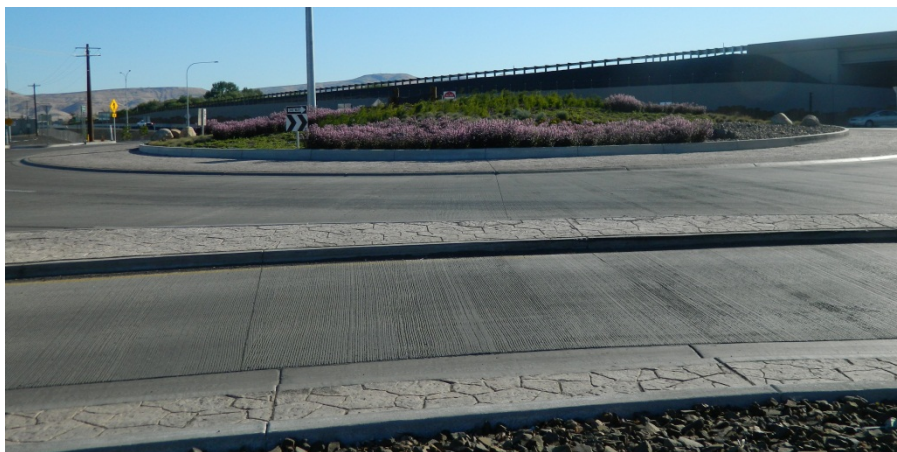
Gently mounded roundabout and concrete color and texture on splitter islands.
