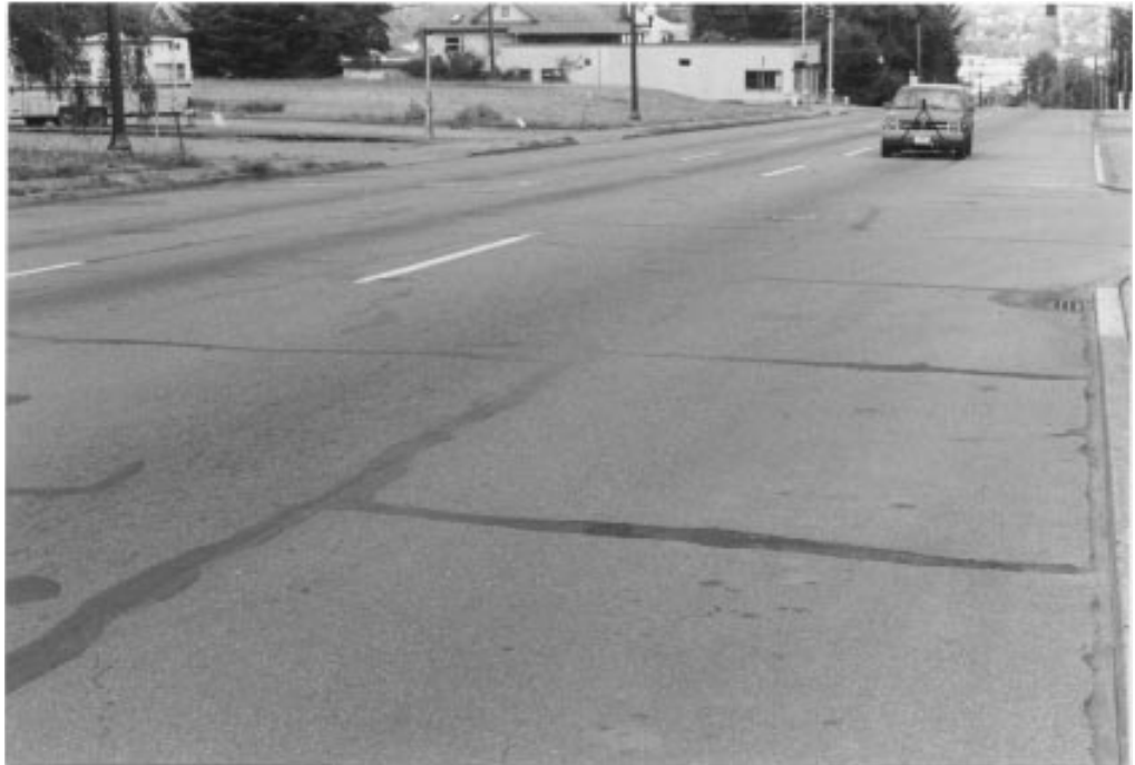
The crack sealing on this local access roadway has been completed.
