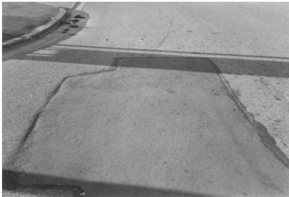
Patching is another commonly used pavement maintenance or rehabilitation activity.
