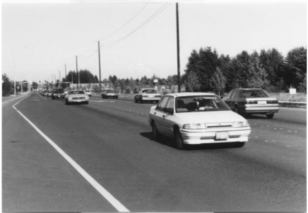
A roadway's lifespan is directly related to the ADT (above) and the percentage of trucks (on the following page) using it.
