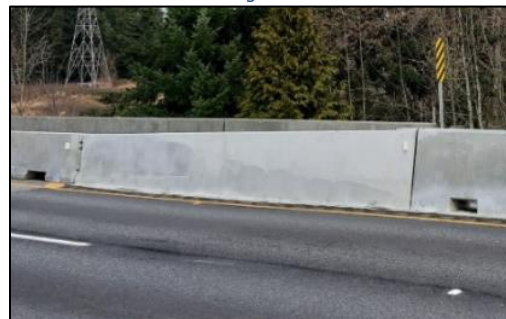
Photo D: Mitigation Strategy - Type F to Single Slope Transition (Height & Shape)
