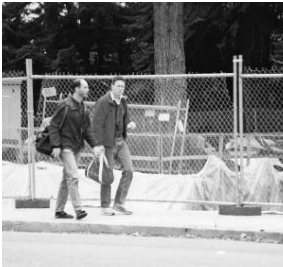
Fencing used to secure a work area supported by blocks needs to be positioned to avoid creating obstacles or tripping hazards for pedestrians.
