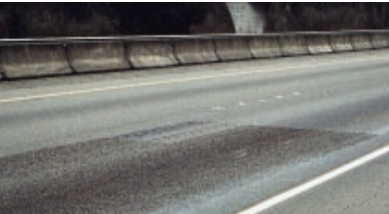
Chip Seal Repair Low
