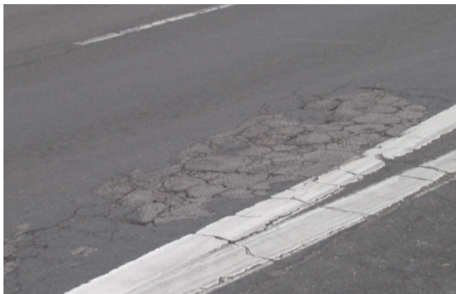
Exhibit 3-3 Alligator Cracking
