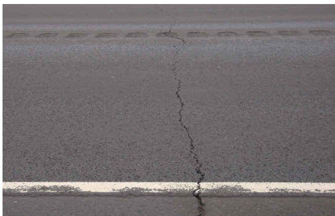
Exhibit 3-2 Transverse Cracking
