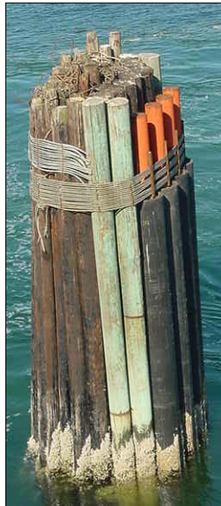
Figure 14 Typical Timber Dolphin
