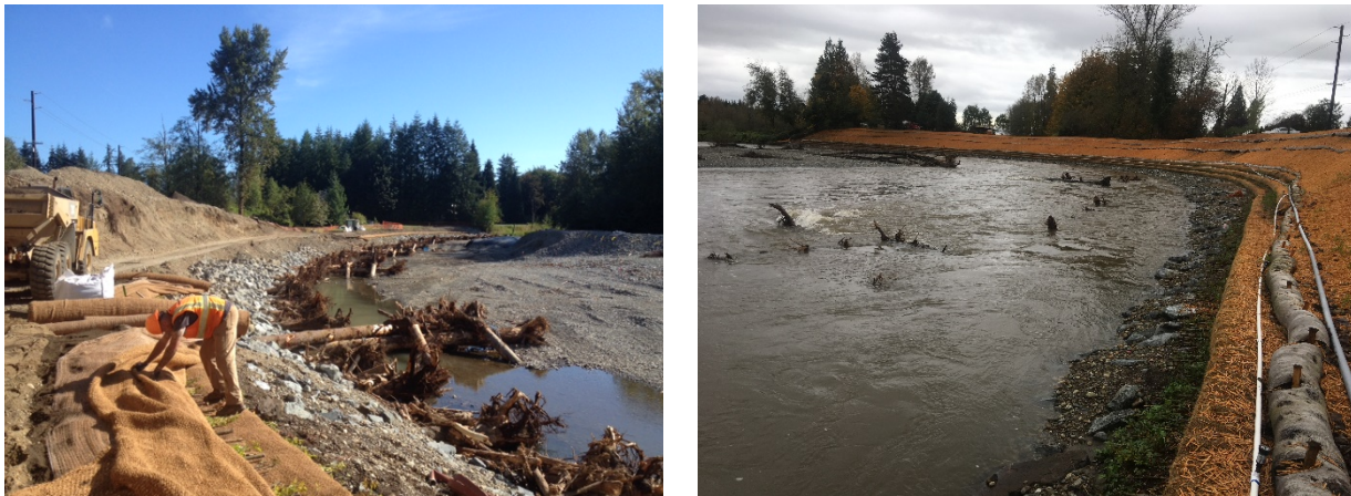
Exhibit 13: SR 92 Pilchuck River Chronic Environmental Deficiency Repair – constructing bank protection and bank protection during first storm.
