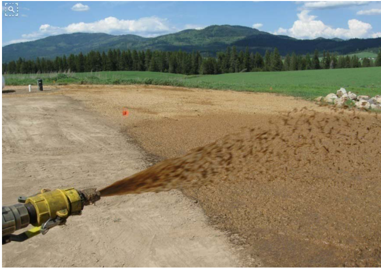
Exhibit 10: Application of hydromulch for erosion control.
