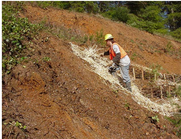
Figure 800. 7 Hand-Distribution of Mulch
