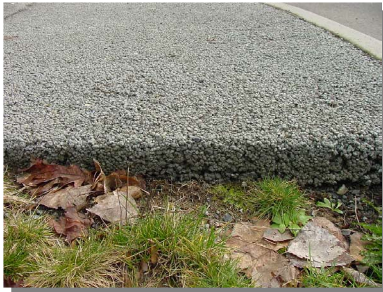
Figure 630.9 Porous concrete sidewalk cross-section, in Olympia
