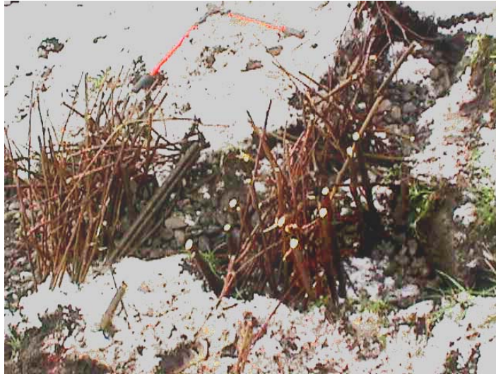
Figure 740.14 Branch Packing in Winter
