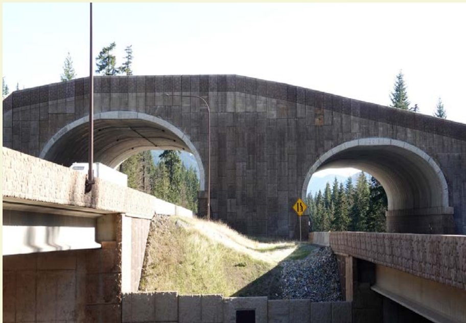
The wildlife bridge crossing on I-90 in Kittitas County reduces the potential for crashes between vehicles and animals on I-90 by providing an unobstructed path between habitats on both sides of the highway.
