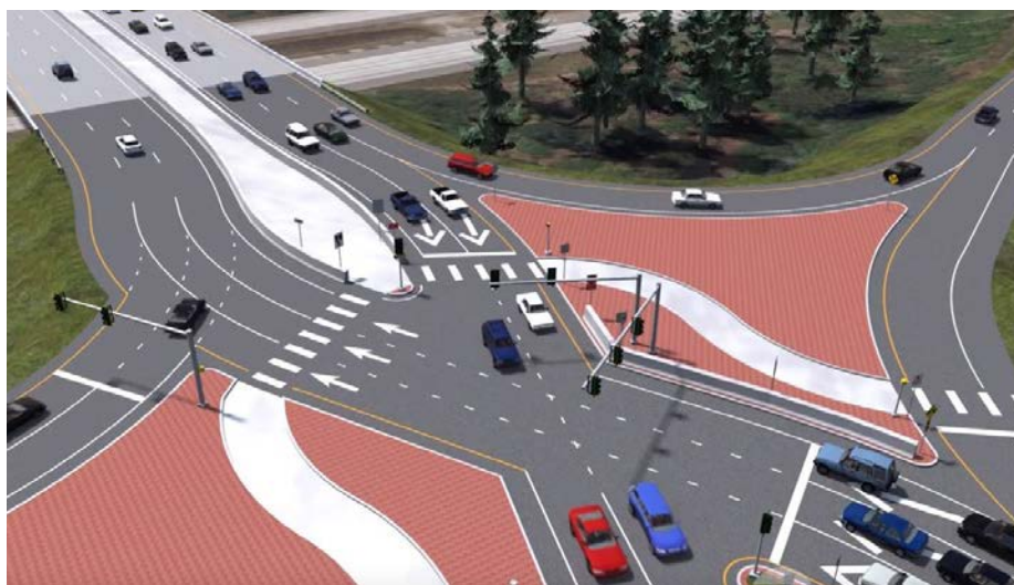
WSDOT is building a diverging diamond interchange ahead of major development in Lacey north of I-5 to ease traffic congestion and reduce the potential for crashes. The $45.9 million I-5 - SR 510 Interchange - Reconstruct Interchange project is the first of its kind in Washington and will reduce conflict points from 26 to 14 for drivers as well as active transportation users. It is scheduled to be completed in winter 2020. A rendition of the south side of the interchange is pictured above.
