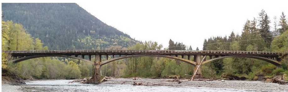
The US 101 bridge over the Elwha River, west of Port Angeles. The Elwha River Bridge needs to be replaced due to bridge scour, which occurs when high volumes of water cause soil erosion around foundations. Foundation scour is the leading cause of bridge failure in Washington and nationwide.
