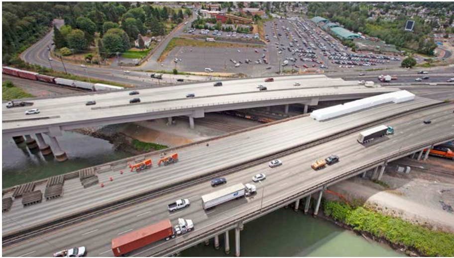
The I-5 Puyallup River bridges are examples of structures that WSDOT will address through its bridge seismic retrofit program. The bridge's columns have hollow cores which were originally constructed in the 1960s and are more vulnerable to earthquake damage than those with solid columns. The existing bridges are being replaced as part of the I-5 HOV project through Tacoma.
