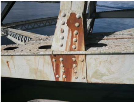
A corroded member on the Julia Butler Hansen steel bridge, which connects Cathlamet to Puget Island in Wahkiakum County. A painting contract for this bridge is nearly complete.
