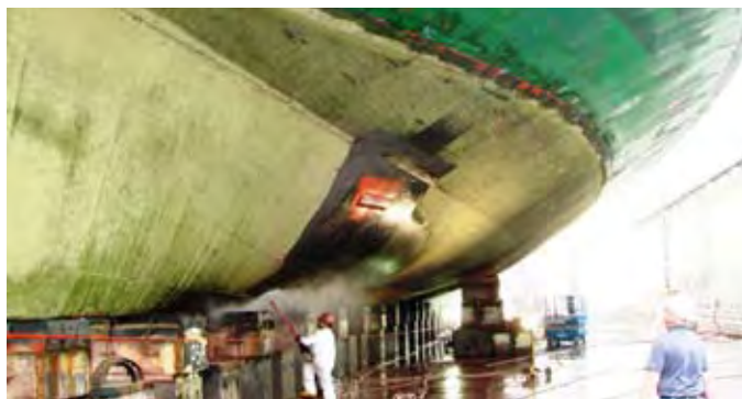
A Steel Electric ferry being prepped for repair work in dry dock in Seattle
