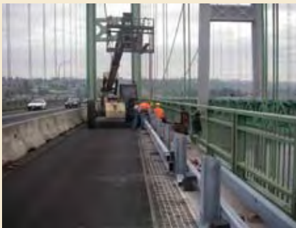
Crews install the new guardrail on the south side of the 1950 bridge.
