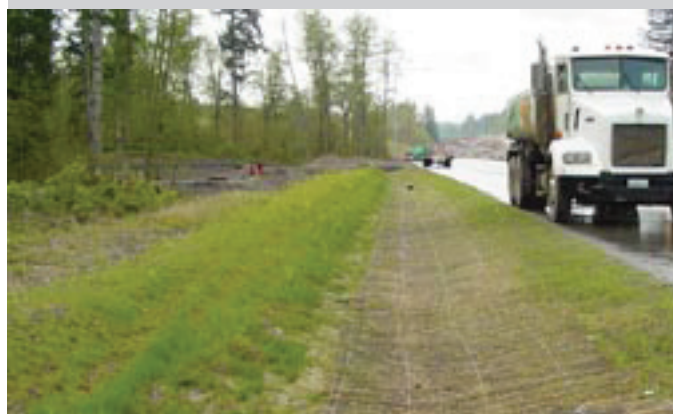
Ecology Embankment on the shoulder of SR 18 filters stormwater runoff before discharging into nearby Jenkins Creek
