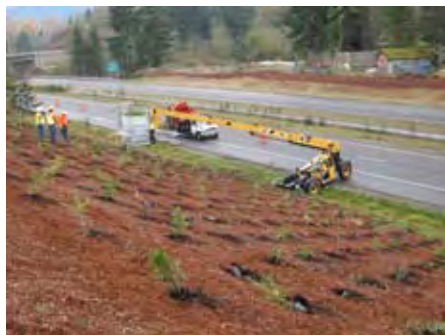
WSDOT is restoring more than 63 acres of roadside affected by the SR 18 widening project
