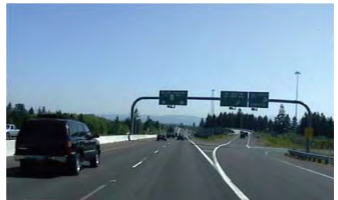
The new interchange on SR 500 in Clark County resulted in a 30% reduction in collisions even with traffic volumes increasing by over 20%
