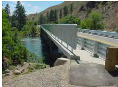
AFTER: The replacement bridge rail meets current safety standards, and greatly reduces the possibility of vehicle penetration.
