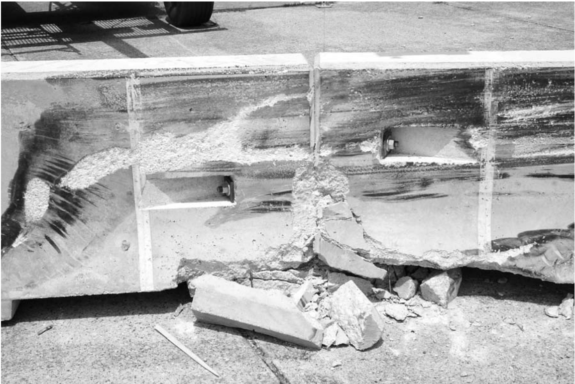
Figure 11. Installation after Test 446924-1.
