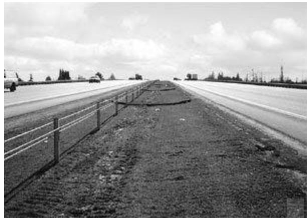
FIGURE 1 Typical cable median barrier installation.
