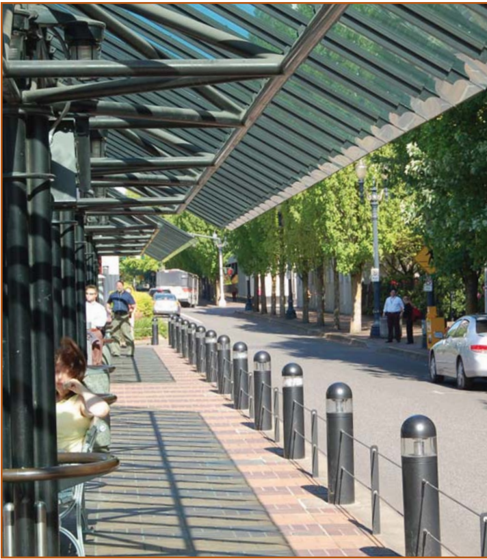
Cable, bollards and distinctive surfaces help define transit, auto and pedestrian areas
