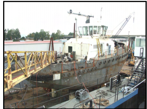
Showing construction of 80' 3800 hp tug in 2004
