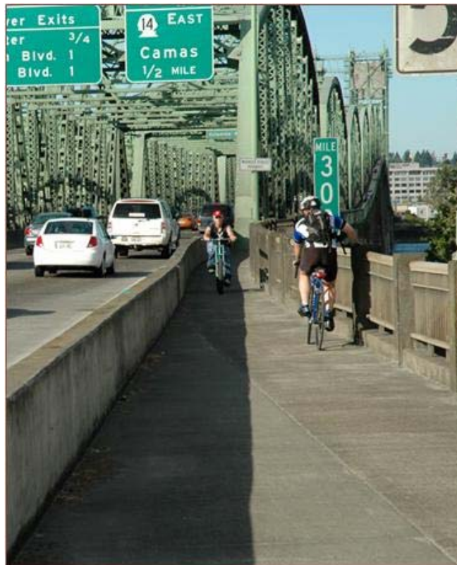
Figure 3-17. Photograph of Existing Non-Standard Multi-Use Pathway
