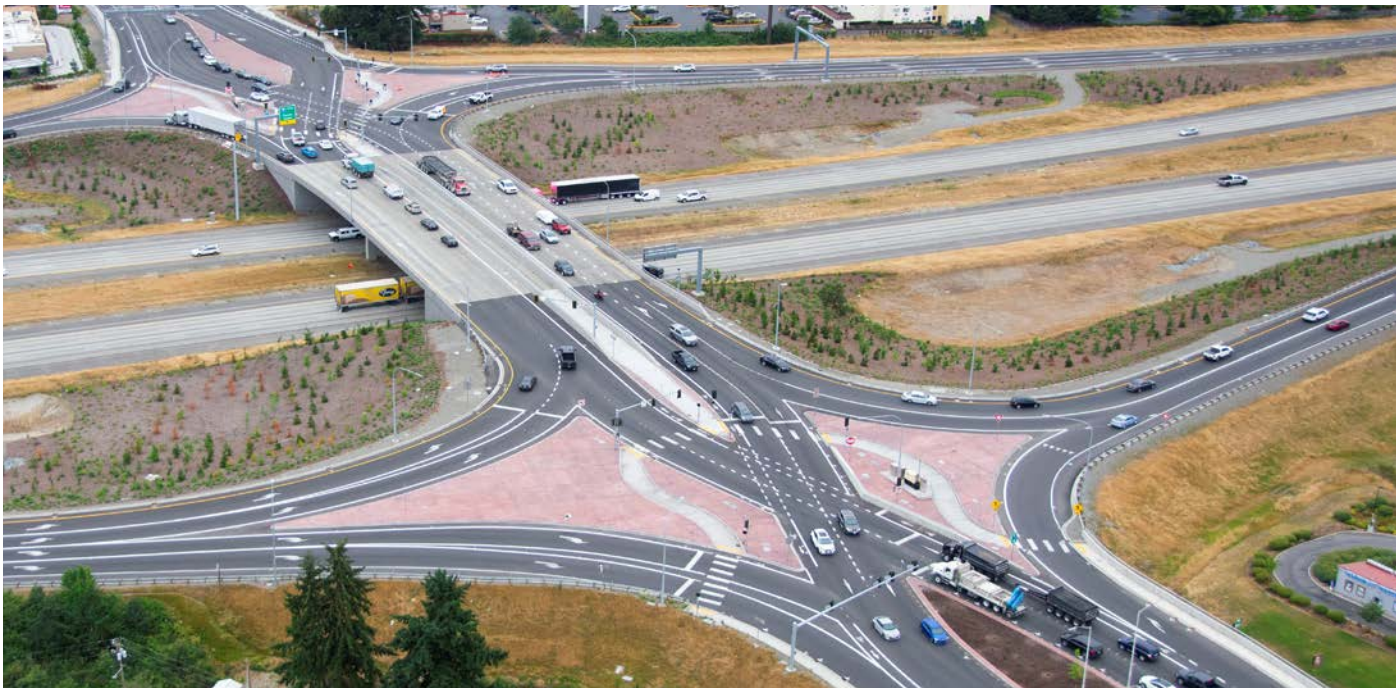
The diverging diamond at SR 510 and Interstate 5 in Lacey is the first of its kind in Washington state. And not only improves traffic flow across the busy intersection but reduces the potential for crashes.
