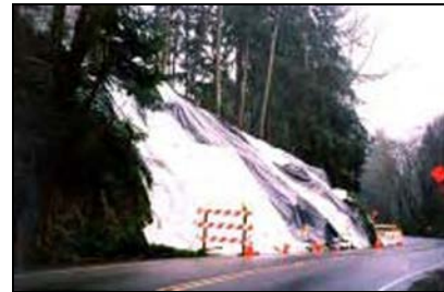
WSDOT may use plastic covering as an erosion control measure.
