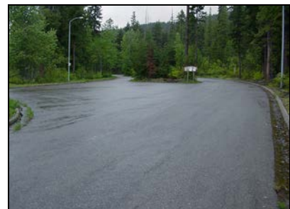
WSDOT will work with USFS and State Parks to mitigate for the loss of the Price Creek Sno-Park (Westbound).
