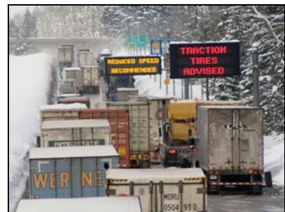
Highway Advisory Radio and variable message signs are an effective way to inform the public of driving conditions and other important information during construction.
