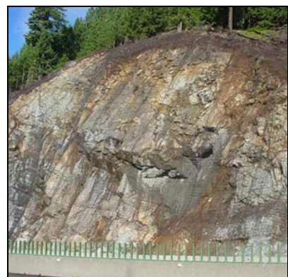
WSDOT may use rock netting at high risk locations throughout the project area.
