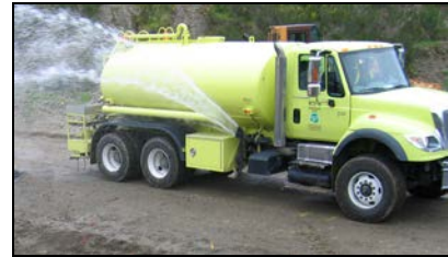
Water wagon wetting down field for dust control.
