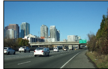
Existing Main Street Overpass
