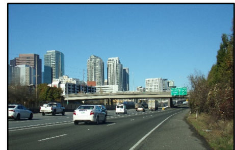
Existing Main Street Overpass
