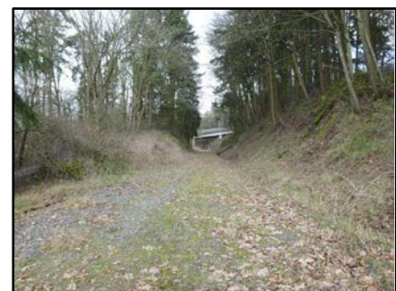
Abandoned segment of the Northern Pacific Railway Lake Washington Beltline
