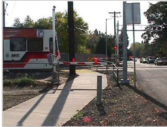
Pedestrian Railroad Warning Device Exhibit 1510-27
