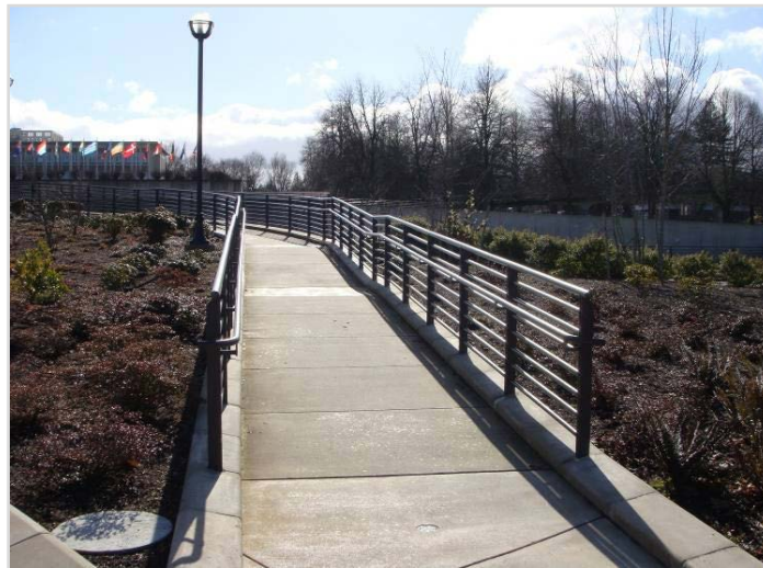
Access Ramp With Accessible Handrails Exhibit 1510-30
