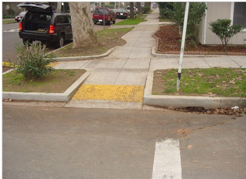
Combination Curb Ramps Exhibit 1510-13
