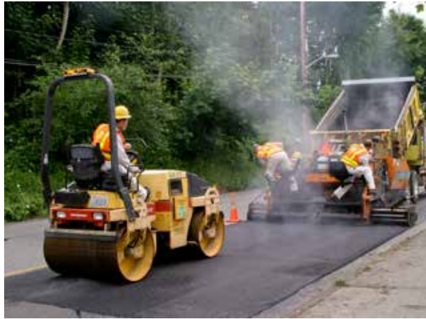
SR 7 Paving Project
