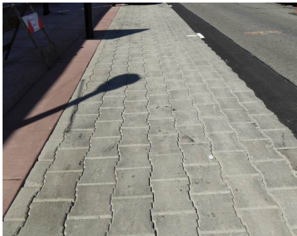
Figure 26. PaveDrain® system installation on Main Street. (Photo courtesy of Joe Mahoney, UW)
