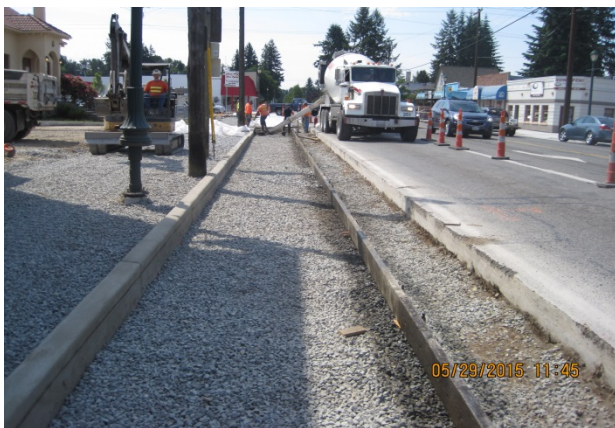
Figure 14. Forms in place on Lewis Street for the parking strips. (Photo courtesy of City of Monroe)
