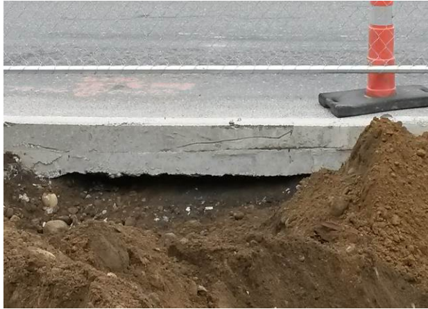
Figure 22. Void space under SR 203.
