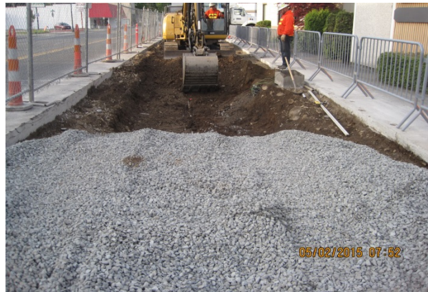
Figure 7. Excavation of subgrade and placement of permeable ballast. (Photo courtesy of City of Monroe)
