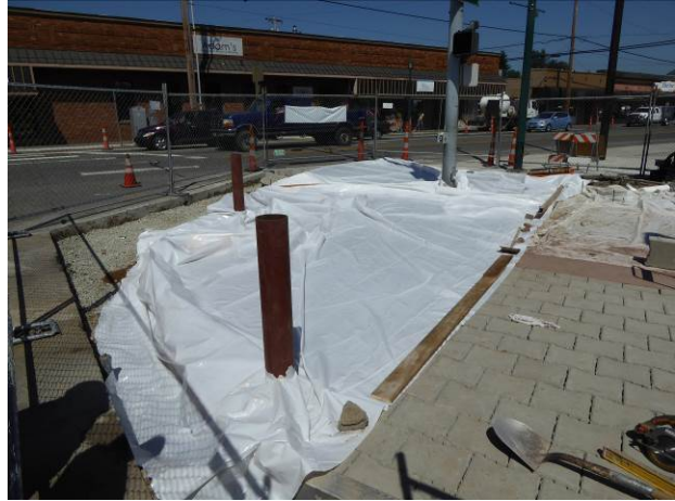
Figure 13. Plastic sheeting used to cure the pervious concrete for 10 days. (Photo courtesy of Joe Mahoney, UW)
