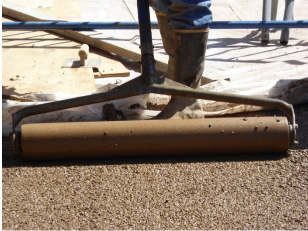
Figure 12. Roller used to smooth the surface of the pervious concrete. A tool release agent was sprayed on the mix prior to rolling. (Photo courtesy of Joe Mahoney, UW)
