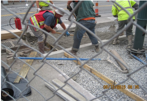
Figure 16. Distributing the pervious concrete in the forms with rakes and shovels. (Photo courtesy of City of Monroe)
