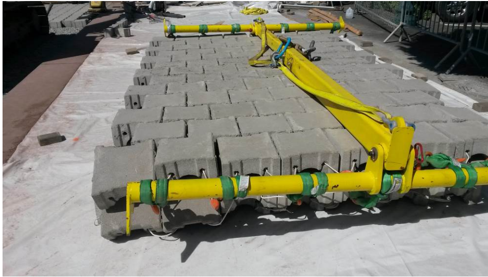
Figure 24. PaveDrain ® mat with lifting gear. (Photo courtesy of Joe Mahoney, UW)
