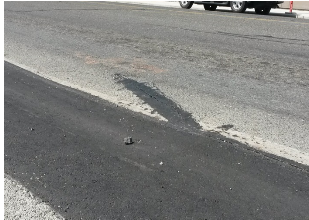
Figure 23. Sealed crack in HMA on SR 203.
