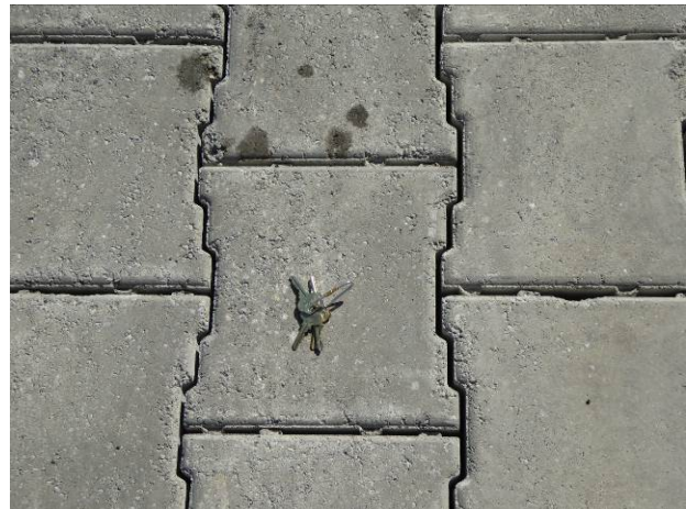
Figure 27. Close-up of PaveDrain® system. (Photo courtesy of Joe Mahoney, UW)
