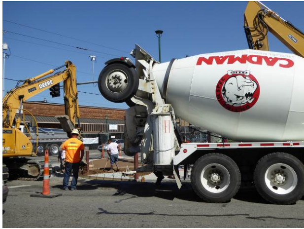
Figure 8. Cadman ready mix truck delivering pervious concrete. (Photo courtesy of Joe Mahoney, UW)
