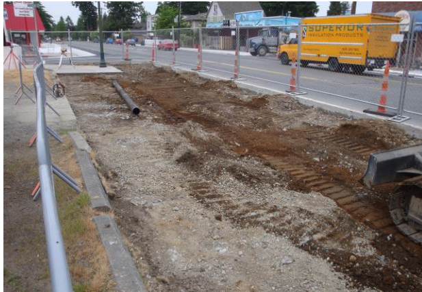
Figure 4. Subgrade on Lewis Street. (Photo courtesy of City of Monroe)
