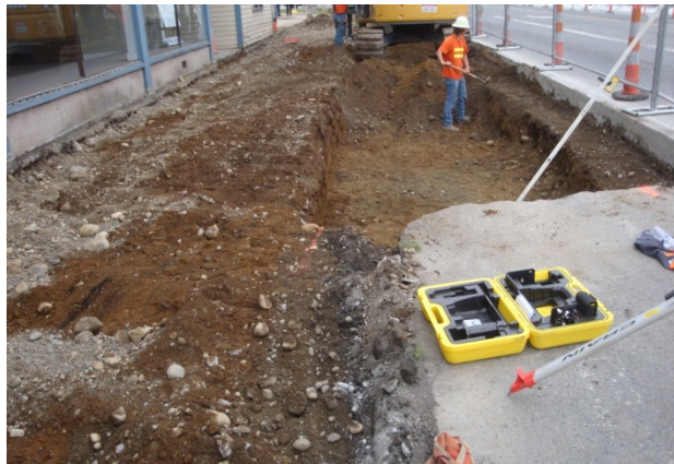
Figure 6. Excavation of subgrade in preparation for the permeable ballast. (Photo courtesy of City of Monroe)
