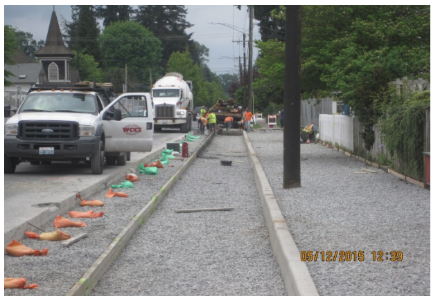
Figure 15. Concrete truck delivering pervious concrete to the forms. (Photo courtesy of City of Monroe)
