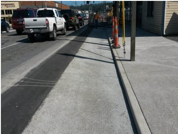
Figure 18. Finished parking strip on Lewis Street. Note HMA filler between SR 203 lane and the parking strip. (Photo courtesy of Joe Mahoney, UW)
