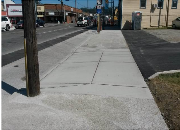
Figure 20. Driveway of dense concrete crossing pervious concrete sidewalk on Lewis Street. (Photo courtesy of Joe Mahoney, UW)
