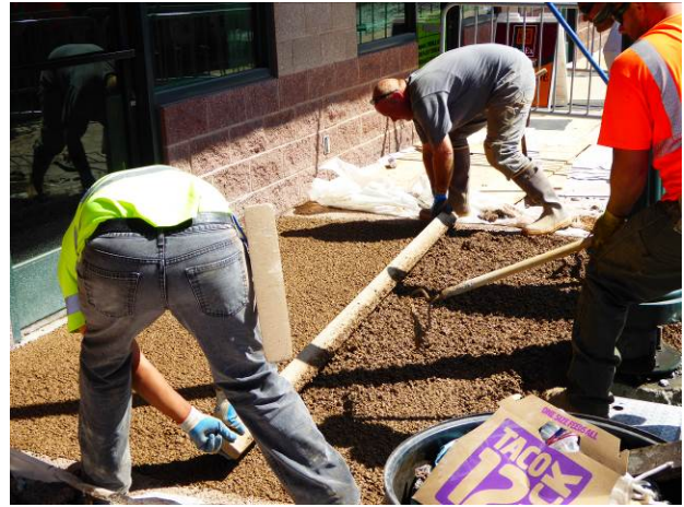
Figure 9. Raking and screeding of delivered concrete. (Photo courtesy of Joe Mahoney, UW)
