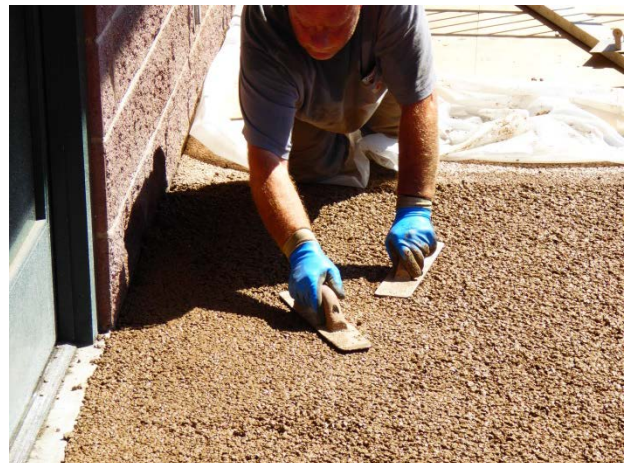
Figure 11. Hand troweling of pervious concrete. (Photo courtesy of Joe Mahoney, UW)
