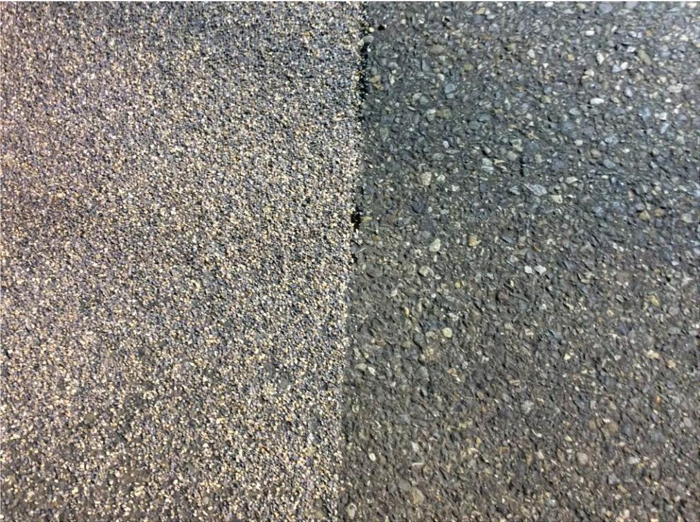
Figure 20. HFST on the left, original HMA on the right, on-ramp to I-90.
