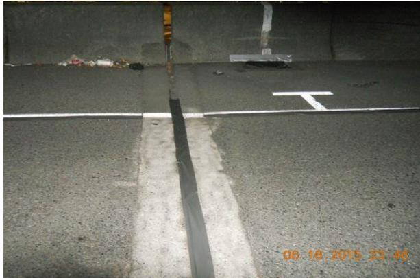
Figure 5. Taped expansion joint.
