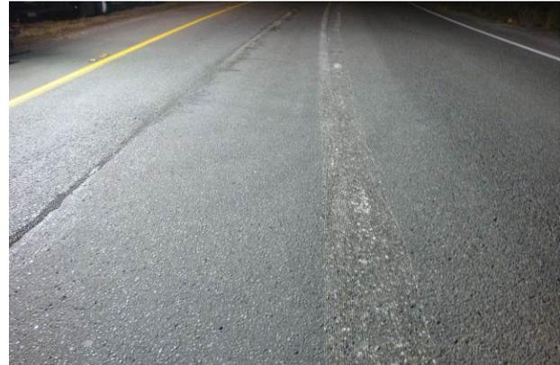
Figure 6. Diamond grinding to remove centerline stripe.
