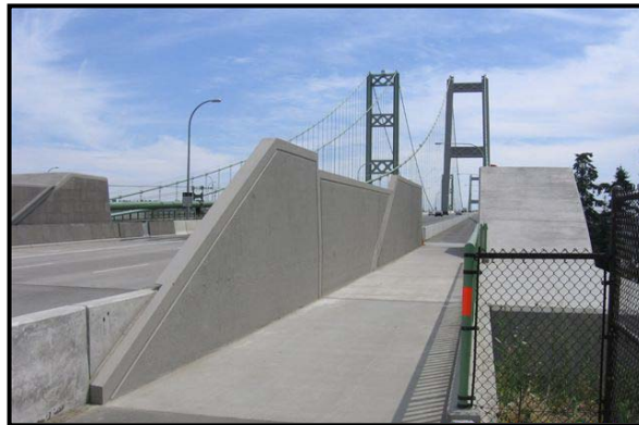
View from behind new wall structure from SW corner of bridge.
