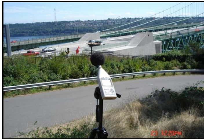
SW bridge corner – pre-construction measurement location with cable housings in background. One of the few sites with a line-of-sight to expansion joint.
