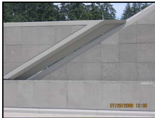
Close up view of sound absorptive panels attached to the new wall structures.
