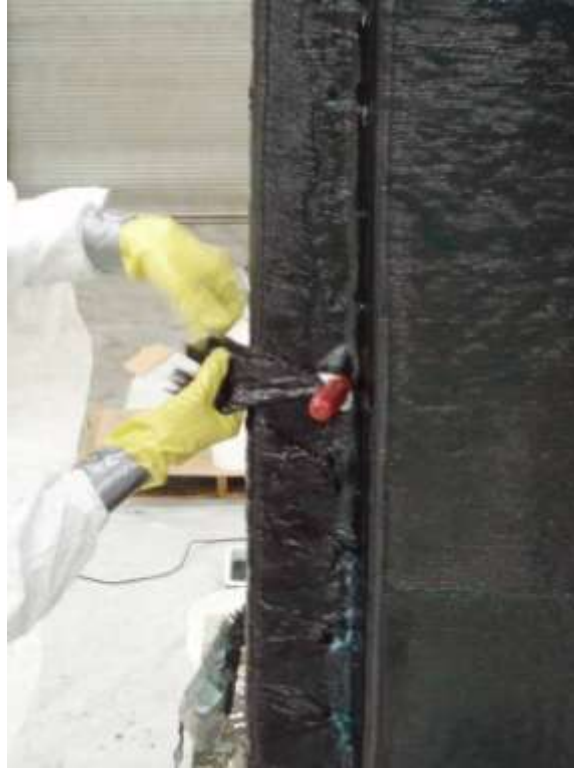
Figure 12 – FRP Anchor Installation
