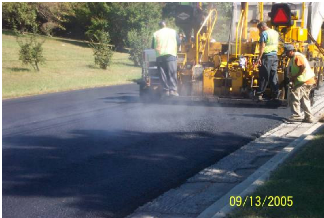
Figure 3.8: Surface course mix with 35% RAP, without Sasobit wax. [24]
