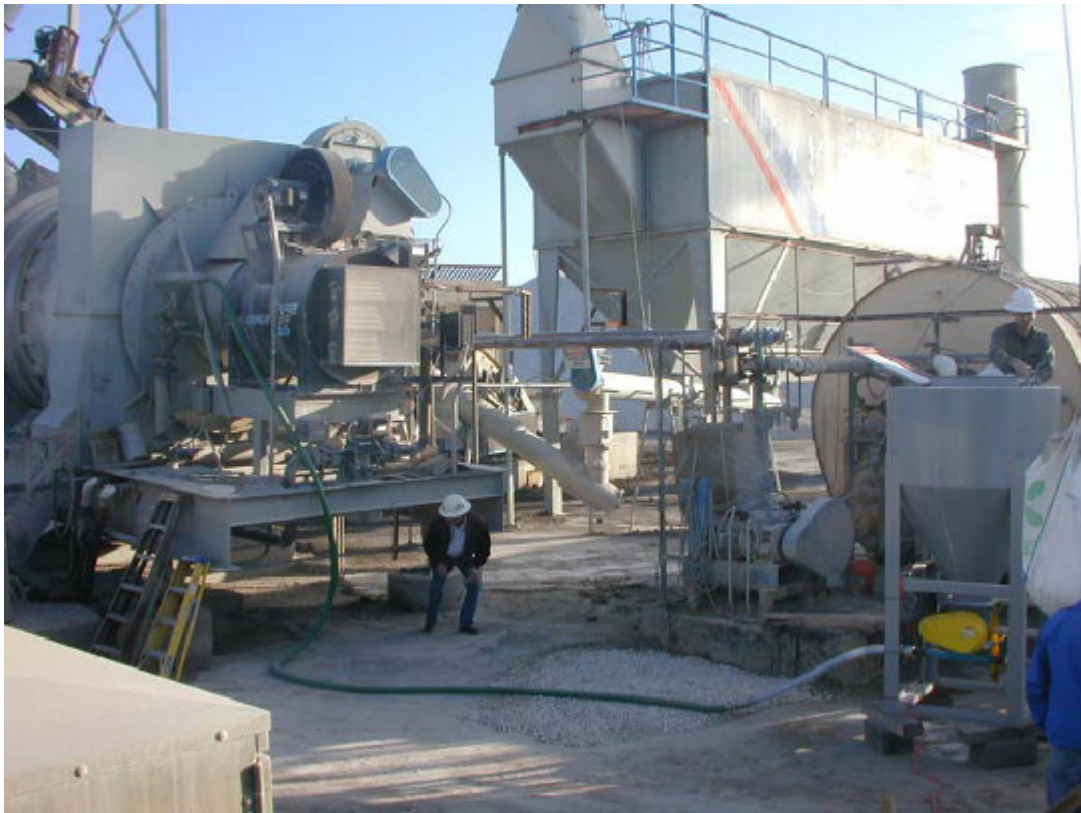
Figure 3.1: Feeder (right) and an existing fiber addition line for Aspha-Min zeolite. [8]
