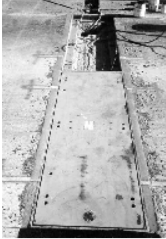
Figure 2-10. Bending plate installation (from Oakridge National Laboratory www.ornl.gov )
