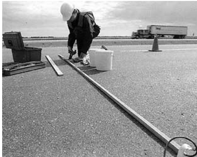
Figure 2-7. Piezoelectric scale layout (from International Road Dynamics Inc., www.irdinc.com )
