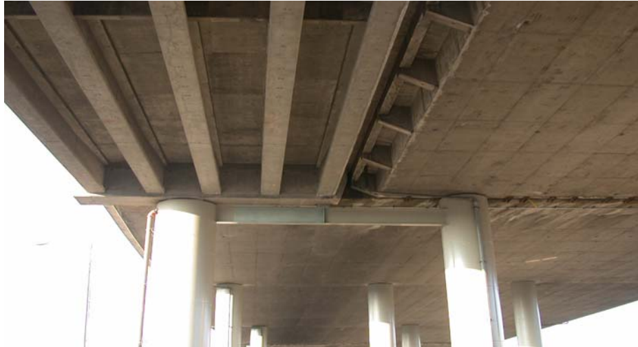
Figure 3-13: Underside of West Off-Ramp
