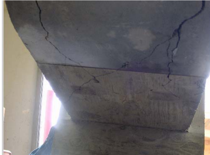
Figure 2-10: Damage to the “Short” Specimen Under Out-of-Plane Loading (Courtesy of Washington State University)
