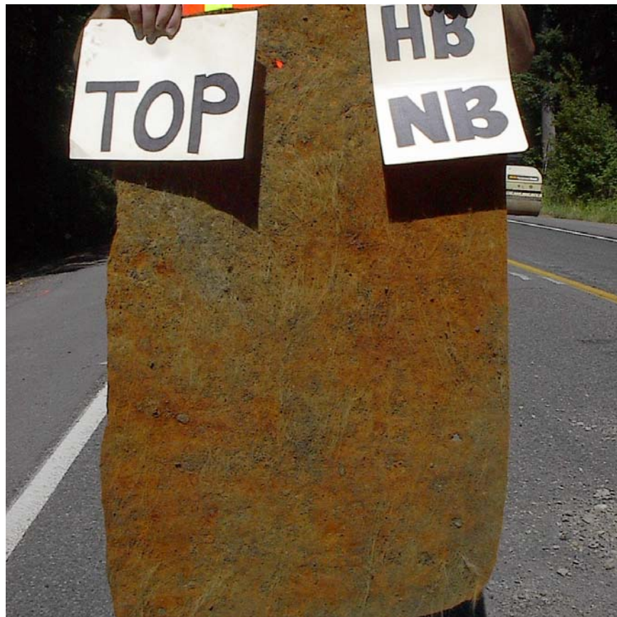
Figure 3.40. Top of HB-NB geotextile after removal.
