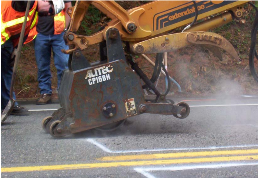
Figure 3.5. Pavement grinding operation.
