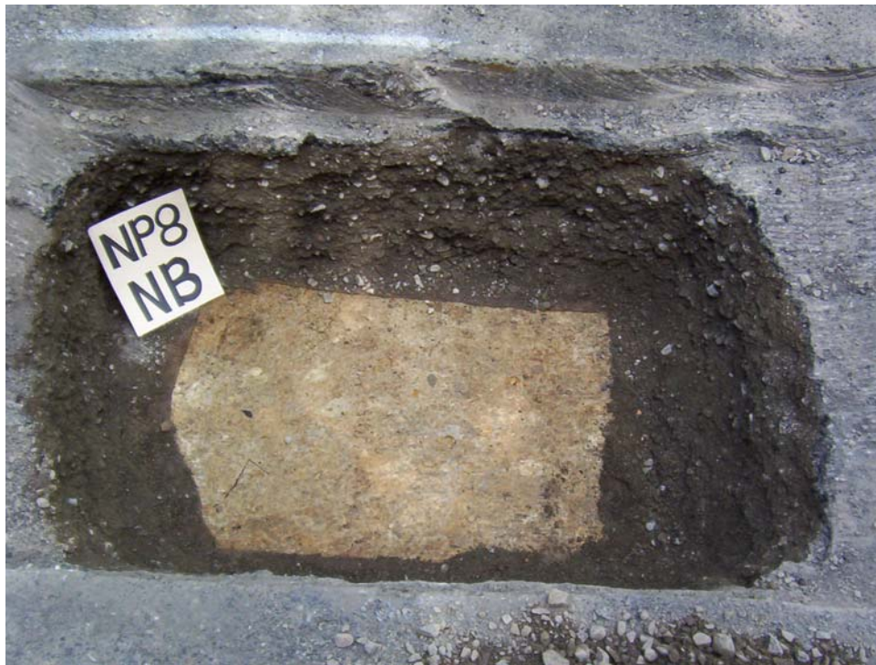
Figure 3.16. NP8-NB test pit after removal of geotextile.
