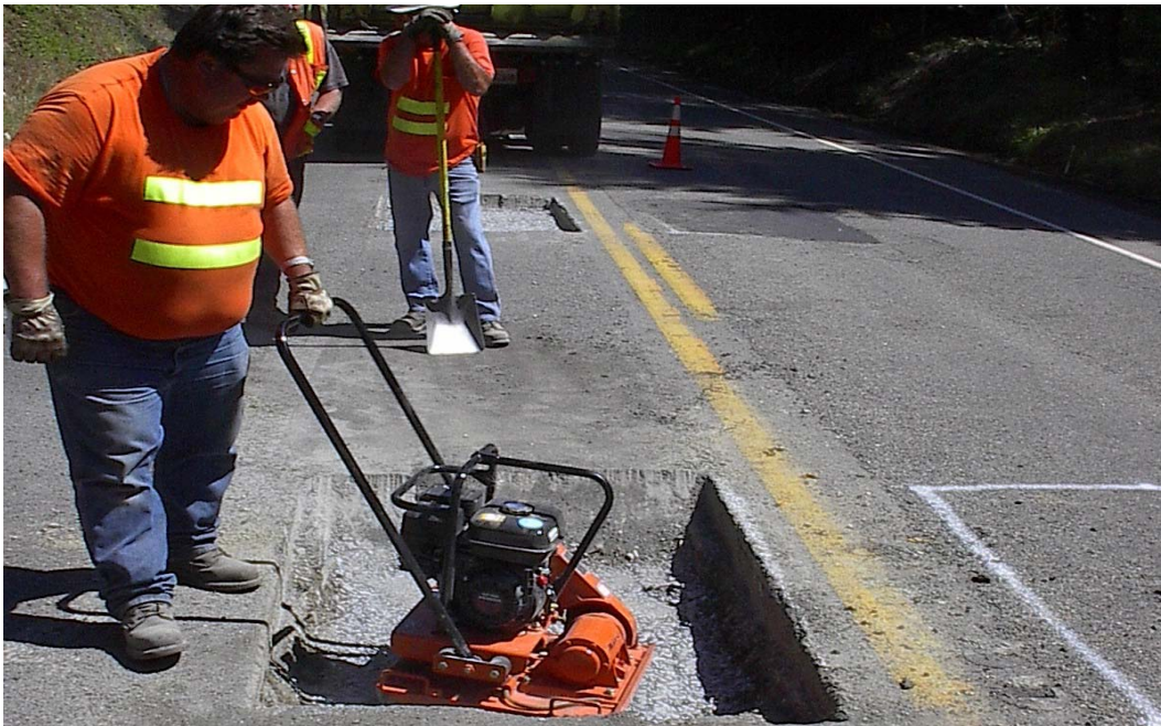
Figure 3.7. Backfill compaction.
