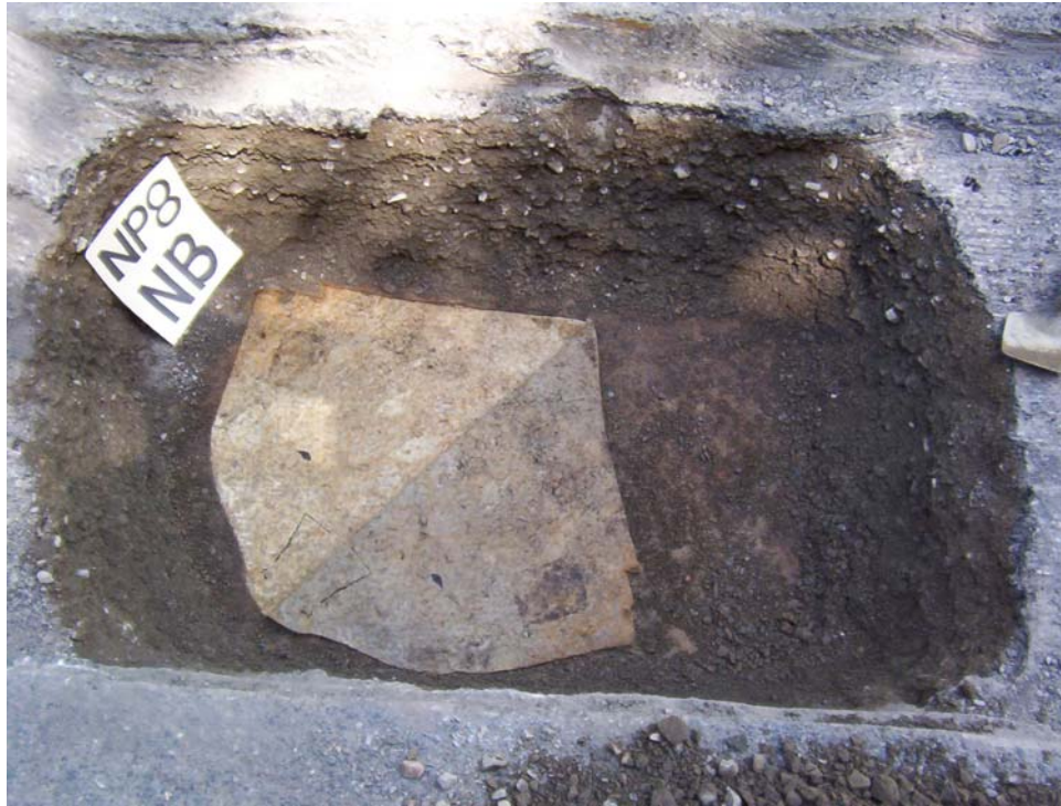
Figure 3.15. NP8-NB test pit with geotextile peeled back.
