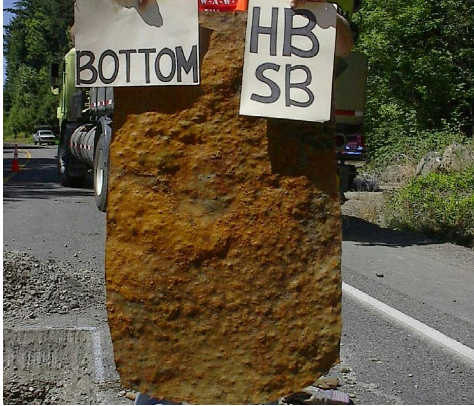
Figure 3.33. Bottom of HB-SB geotextile after removal.
