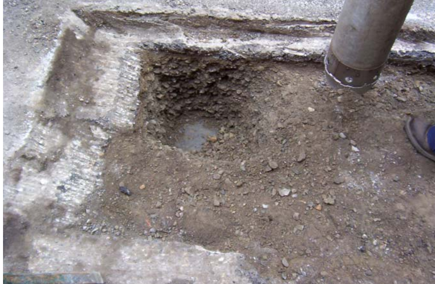
Figure 3.11. First encounter of geotextile in SF-NB test pit.
