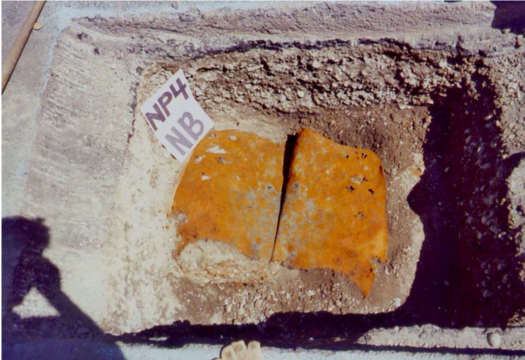
Figure 3.35. NP4-NB test pit with geotextile peeled back.
