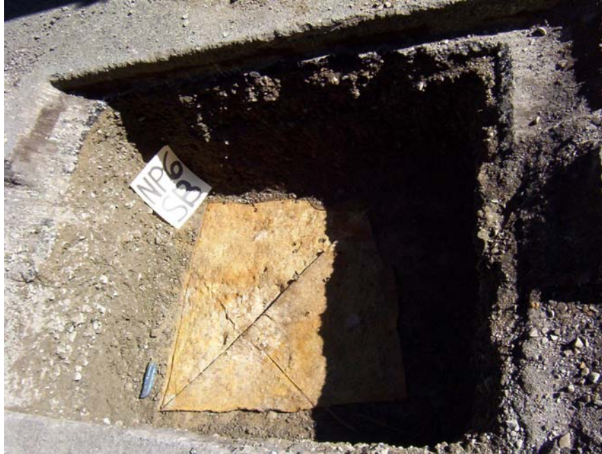
Figure 3.19. NP6-SB test pit with geotextile peeled back.
