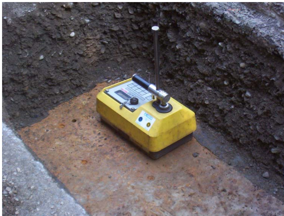
Figure 3.14. Nuclear density test in SF-NB test pit.
