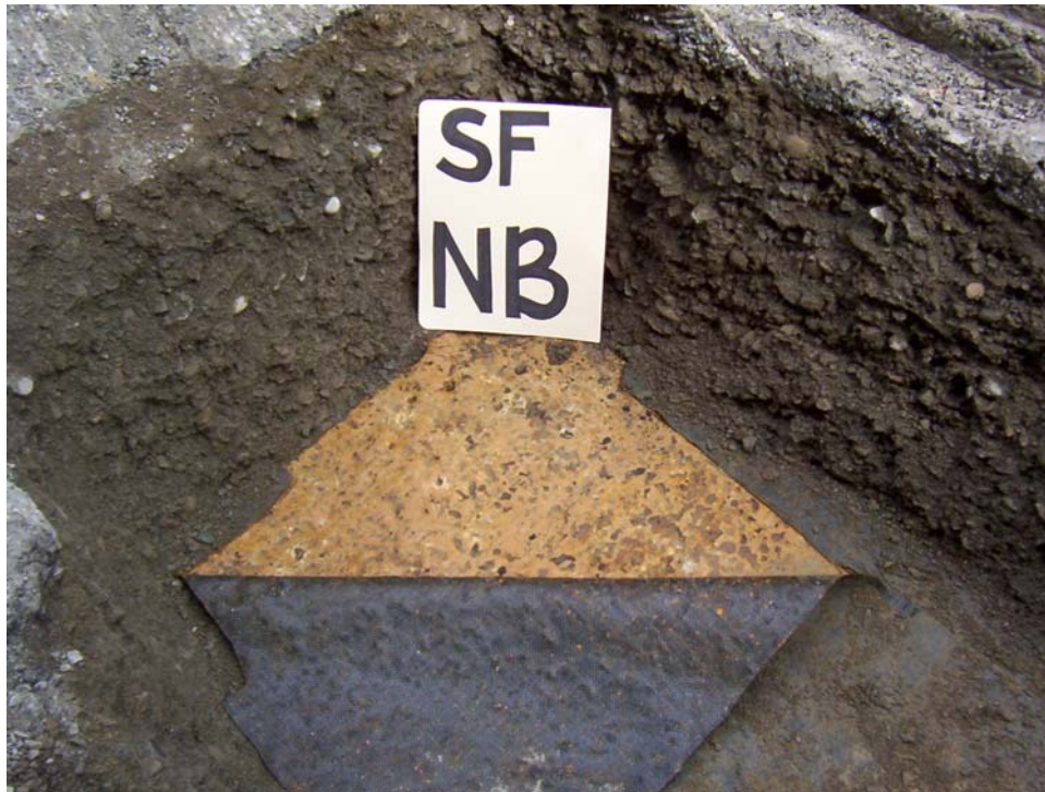
Figure 3.12. SF-NB test pit with geotextile peeled back.
