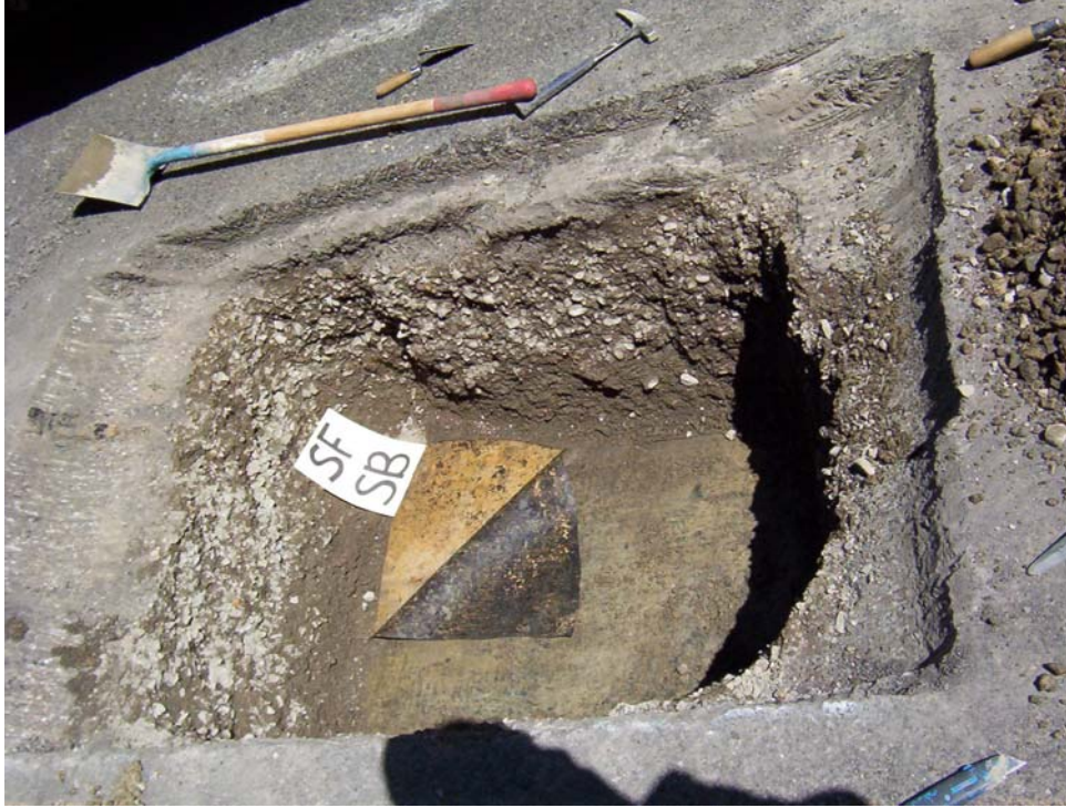
Figure 3.25. Geotextile peeled back in SF-SB test pit.
