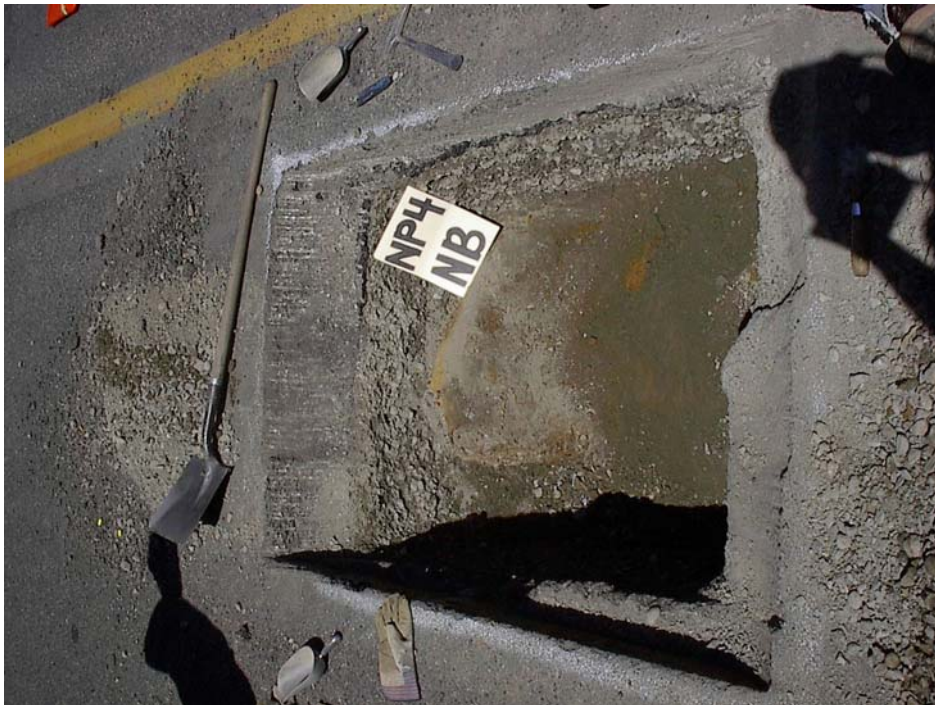
Figure 3.34. NP4-NB test pit prior to geotextile removal.
