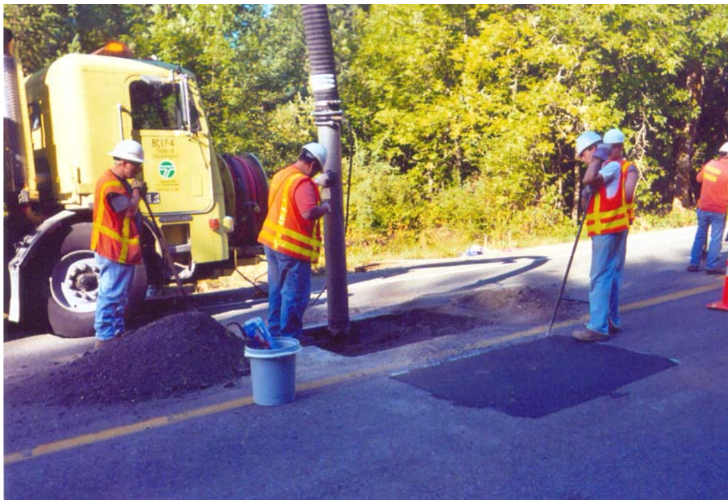
Figure 3.6. Removing the base course with a vacuum truck.
