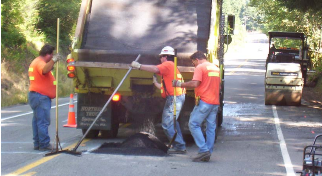
Figure 3.8. Placing a patch over the test pit.
