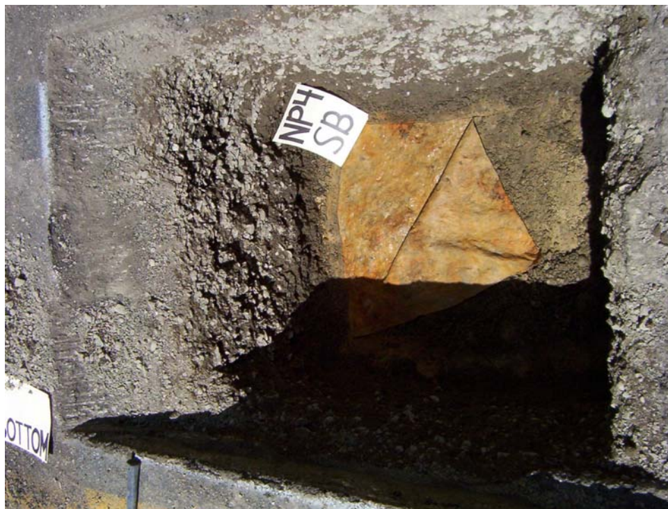
Figure 3.28. NP4-SB test pit with geotextile peeled back.
