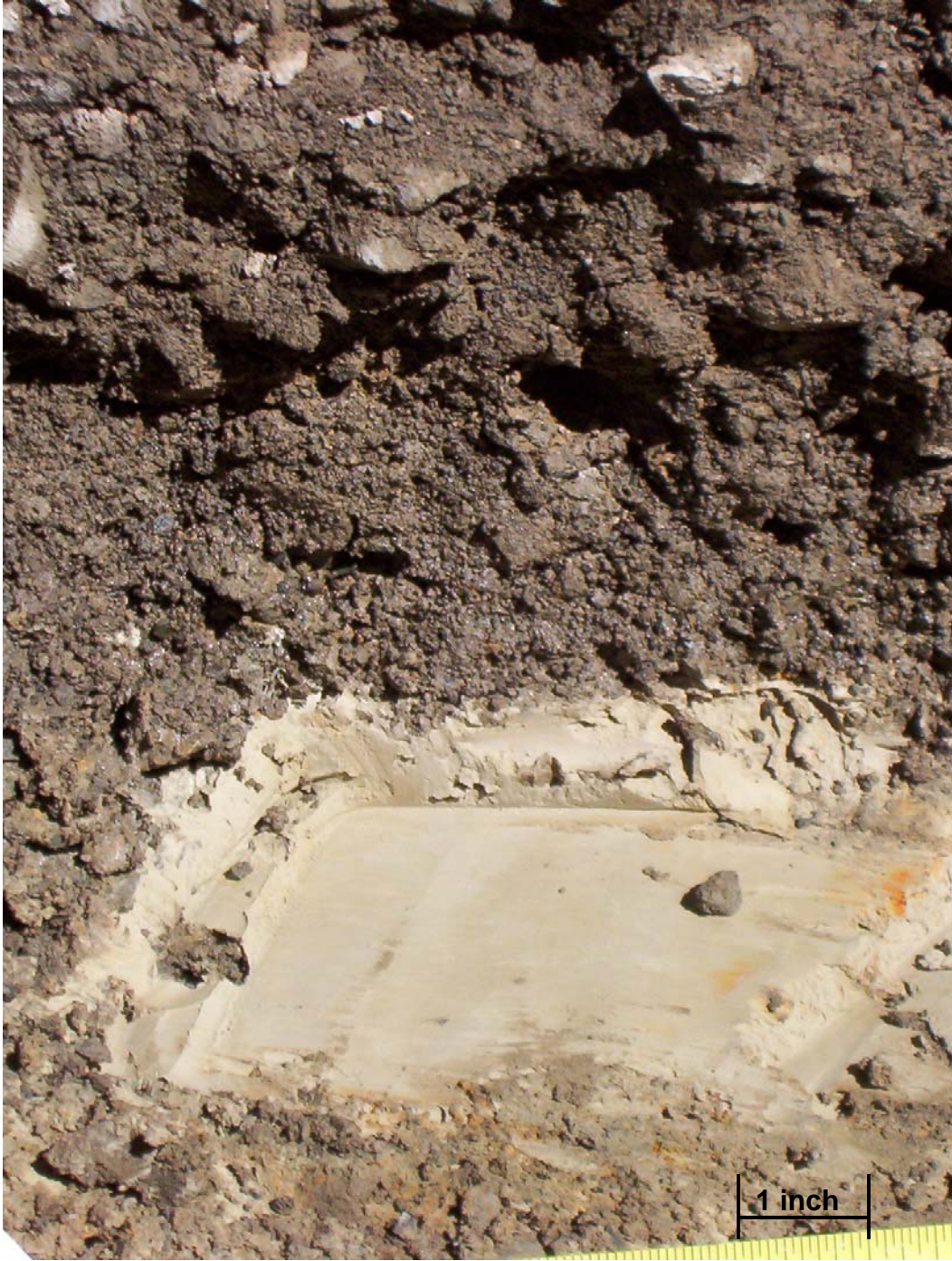
Figure 3.24. Soil-SB test pit after exposure of subgrade.
