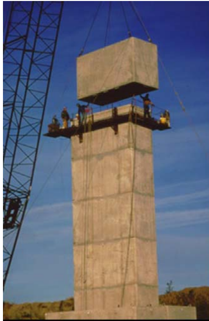
Figure 6.4: Construction of a precast segmental column using match-cast joints (Pate 1995)
