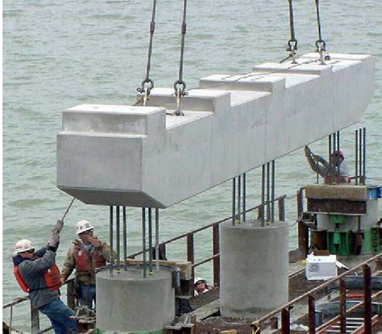
Figure 6.6: Erection of a precast multi-column pier cap-beam (FHWA 2004)
