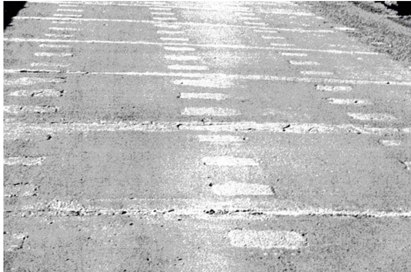
Figure 2.11: Typical surface of a full-depth deck panel bridge without a wearing surface (Issa et al. 1995b)
