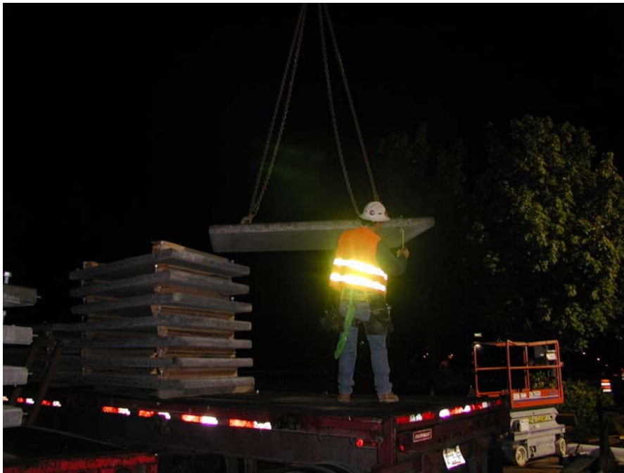
Figure 3.3: Removing panels from a flatbed trailer (Courtesy of WSDOT)
