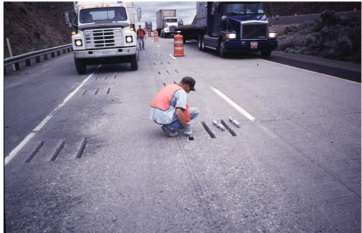
Photo 21. Dowel bar assemblies are placed into slots.
