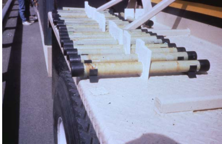
Photo 20. Prepared dowel bars with end caps, chairs and core foam insert.
