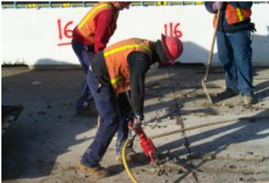
2. Remove existing concrete from slots.
