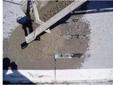
6. Place patching material.
