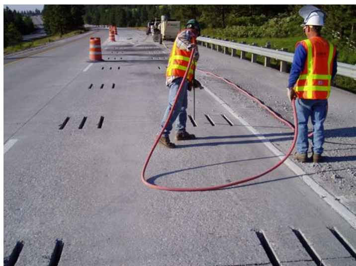
Photo 14. Cleaning slots with compressed air.
