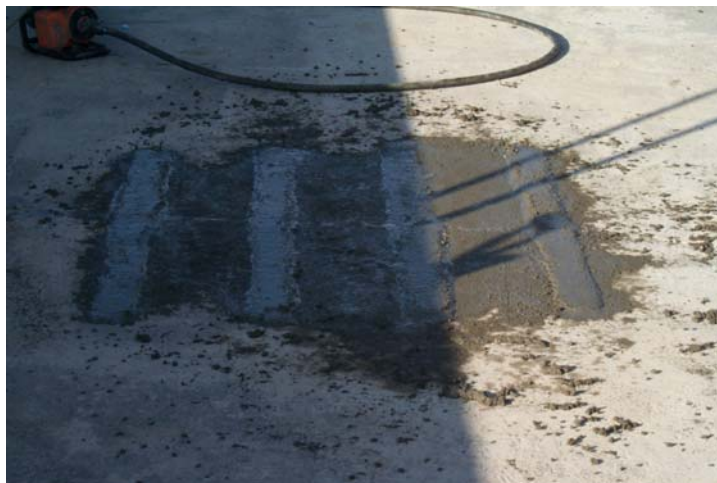
Photo 33. Finished patching material should be left slightly high to minimize fine material at final slot surface.
