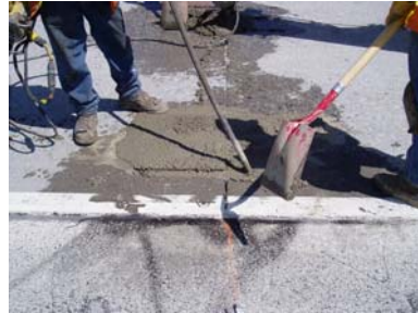
7. Consolidate patching material.
