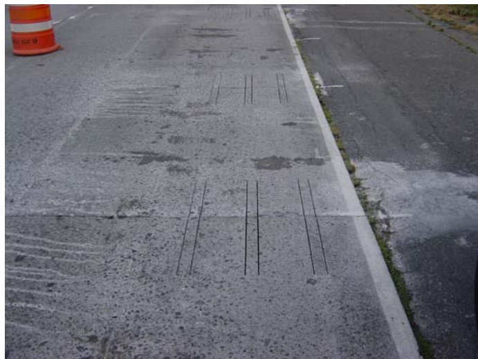
Photo 2. Cut slots, parallel to centerline and perpendicular to transverse (non-skewed) joint.
