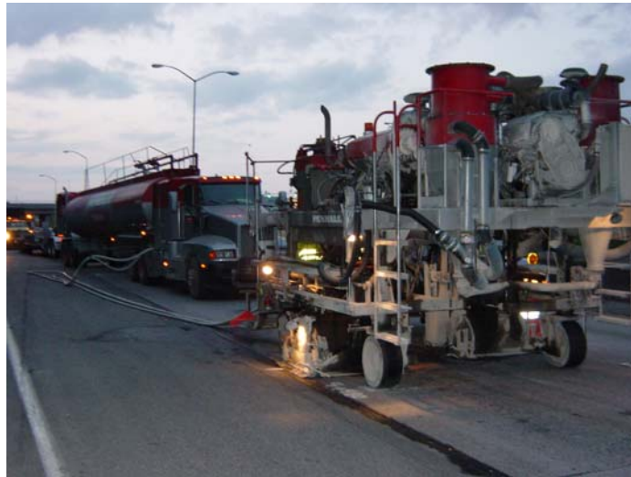
Photo 1. Saw cutting slots.
