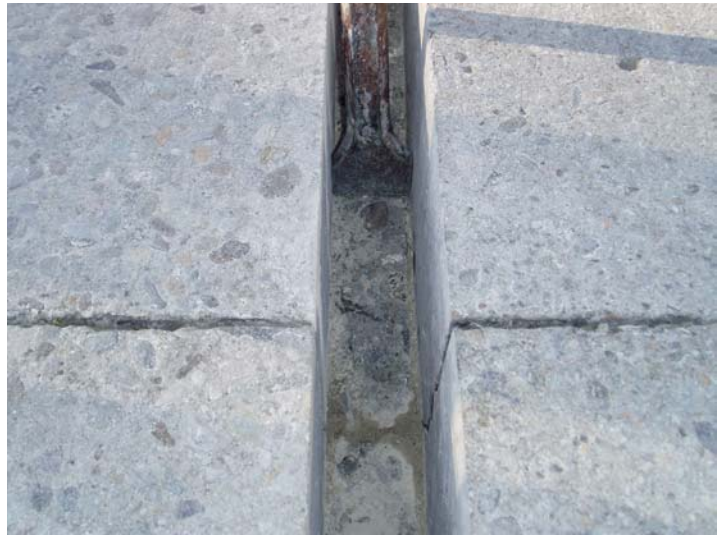
Photo 9. Leveling the bottom of a slot.
