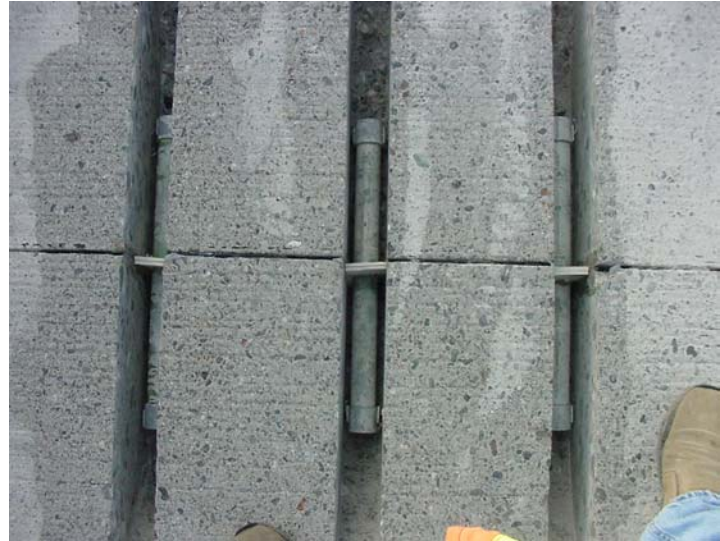
Photo 23. Dowel bar placement and alignment at a transverse joint.
