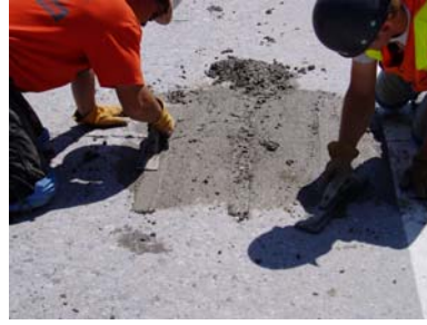
8. Finish patching material.
