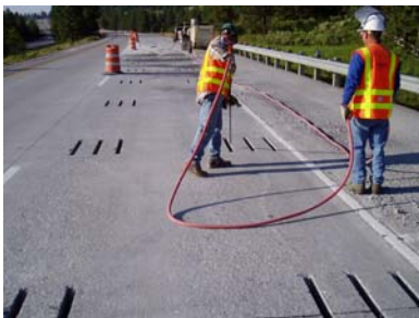
3. Clean slots of all debris.
