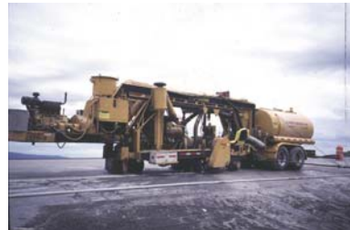
9. Diamond grind pavement surface.
