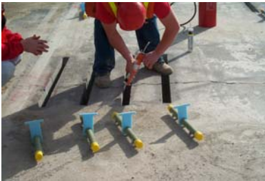
4. Place silicone at all joints/cracks.
