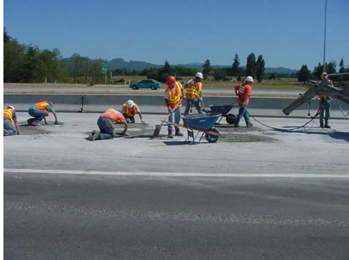
Photo 28. Placing patching material.
