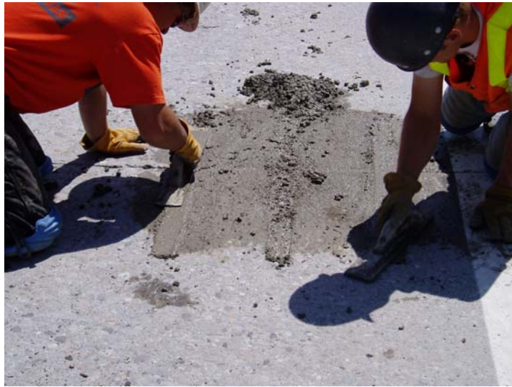
Photo 32. Finishing patching material.
