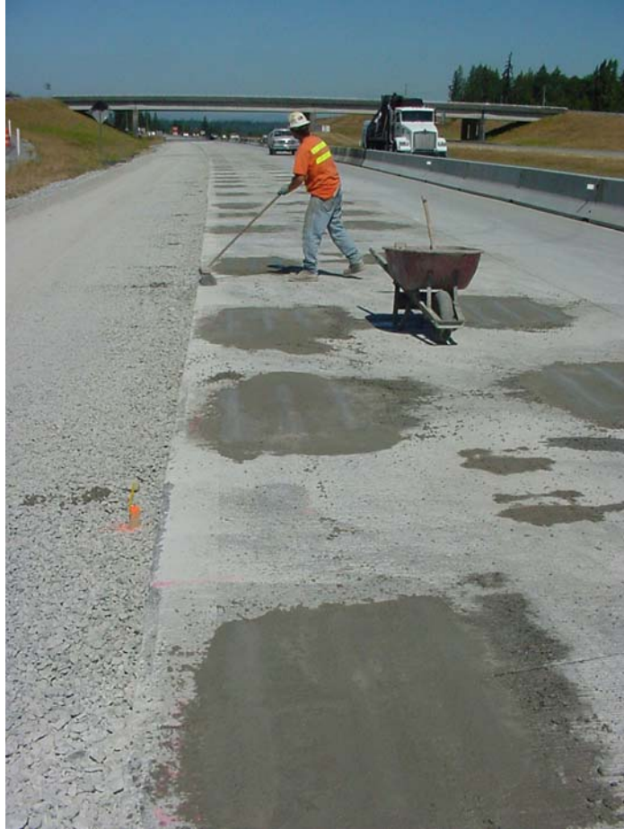
Photo 34. Completed placement of patching material.
