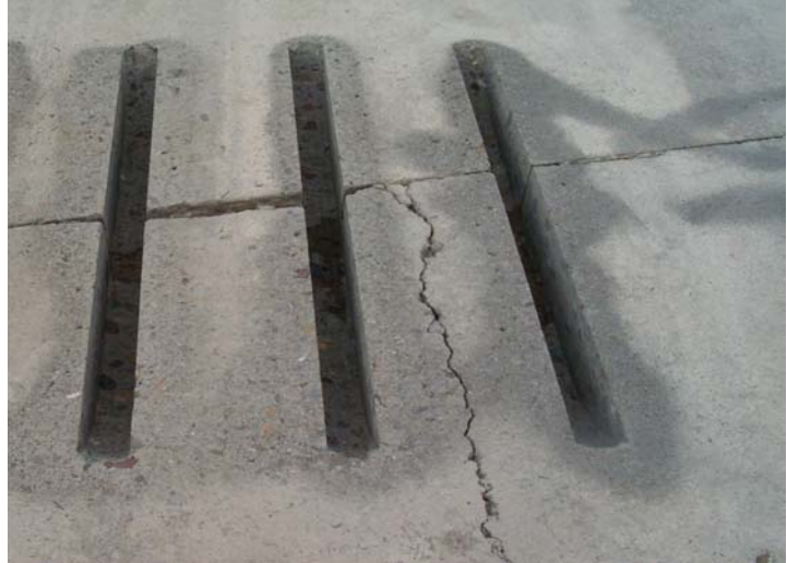
Photo 7. Align dowel bar slots to miss an existing longitudinal crack.
