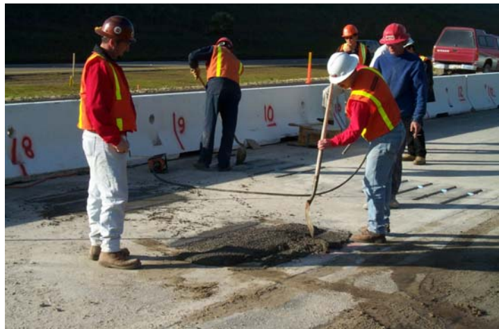
Photo 30. Shoveling patching material into slots.
