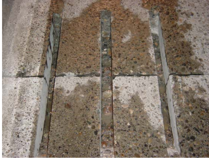
Photo 15. Slots and the surrounding concrete area have been cleaned.
