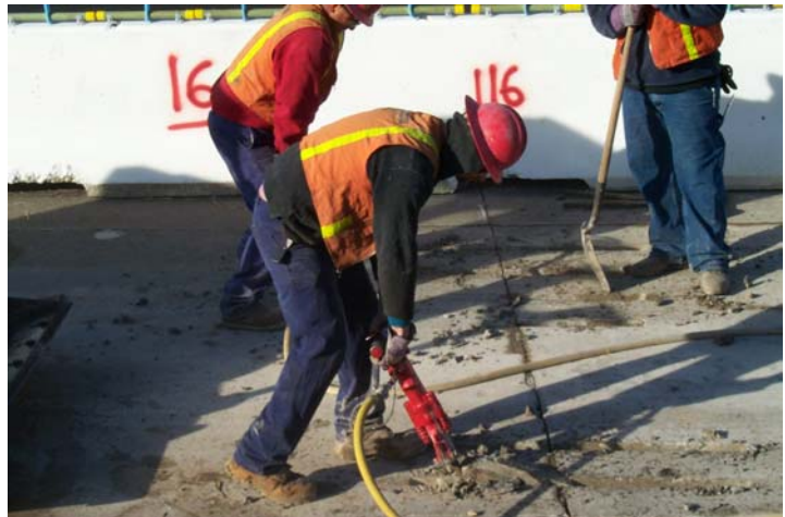
Photo 8. Maintain jackhammer at a 45-degree angle.
