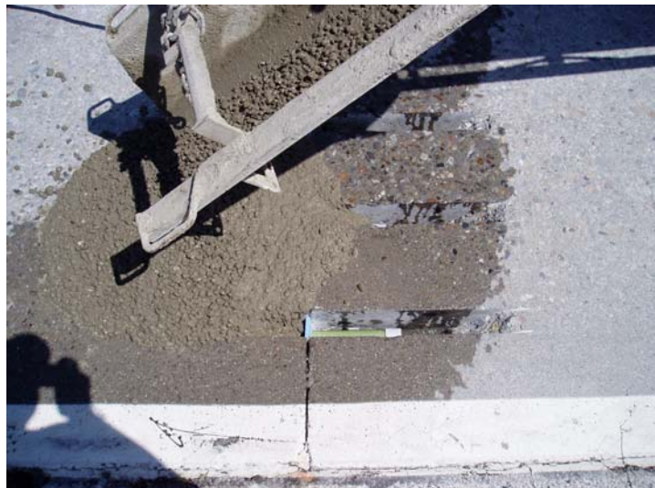
Photo 29. Placing patching material.
