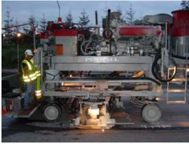
1. Cut dowel bar retrofit slots.
