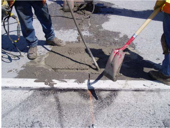
Photo 31. Consolidating patching material.
