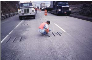
5. Place dowel bar assemblies in slots.
