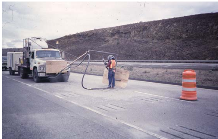
Photo 13. Provide protection to traffic during the sandblasting operation.
