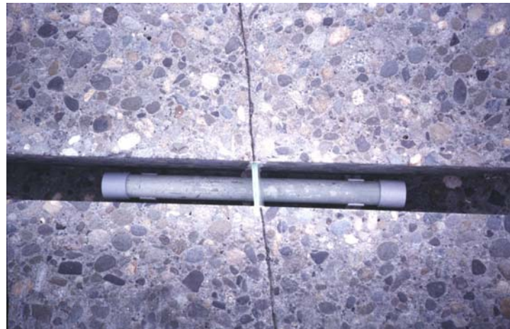
Photo 24. Dowel bar placement and alignment at a skewed transverse joint.
