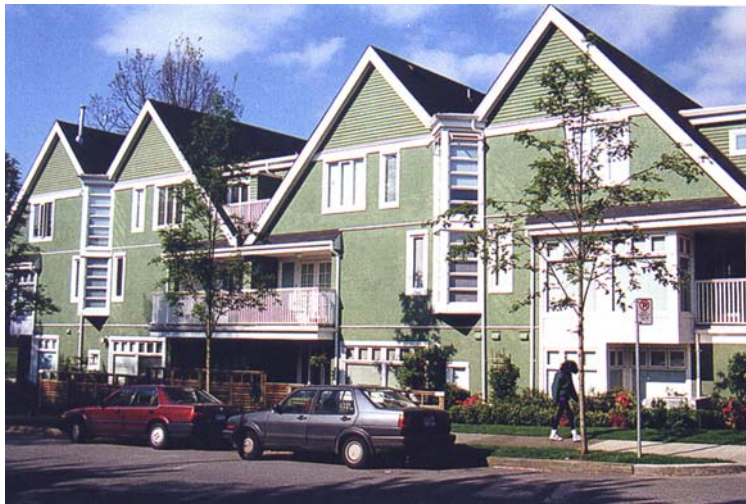
Figure II.5 Townhouse in Vancouver, B.C., with steeply scaled roof form minimizes the apparent bulk of the buildings, and contributes to a single-family appearance.
