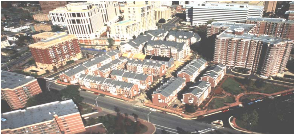
Figure II.2: Considering density at the site level. Combining mixed-use development of different densities in the Courthouse area in Arlington County, Va.
